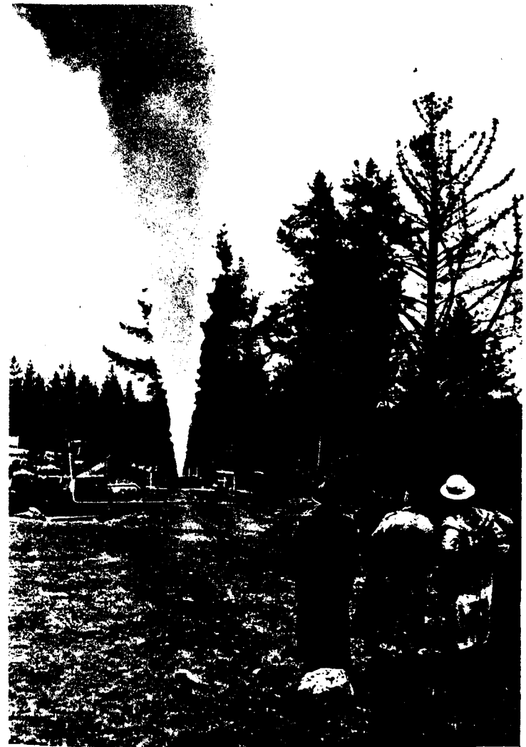
13. Uncapping a test bore in the grounds of the Wairakei Hotel (same area). The requirement for electricity-generation is to obtain 'dry' steam in quantity, the steam from this bore being 'wet'. Natural steam has been used already in the Lardarello district of Tuscany as a source of power.
