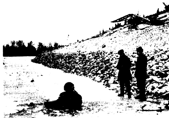
9. Volga-Don navigation canal: watershed section. Inspecting an under-water filter in the canal side (February 1952).
