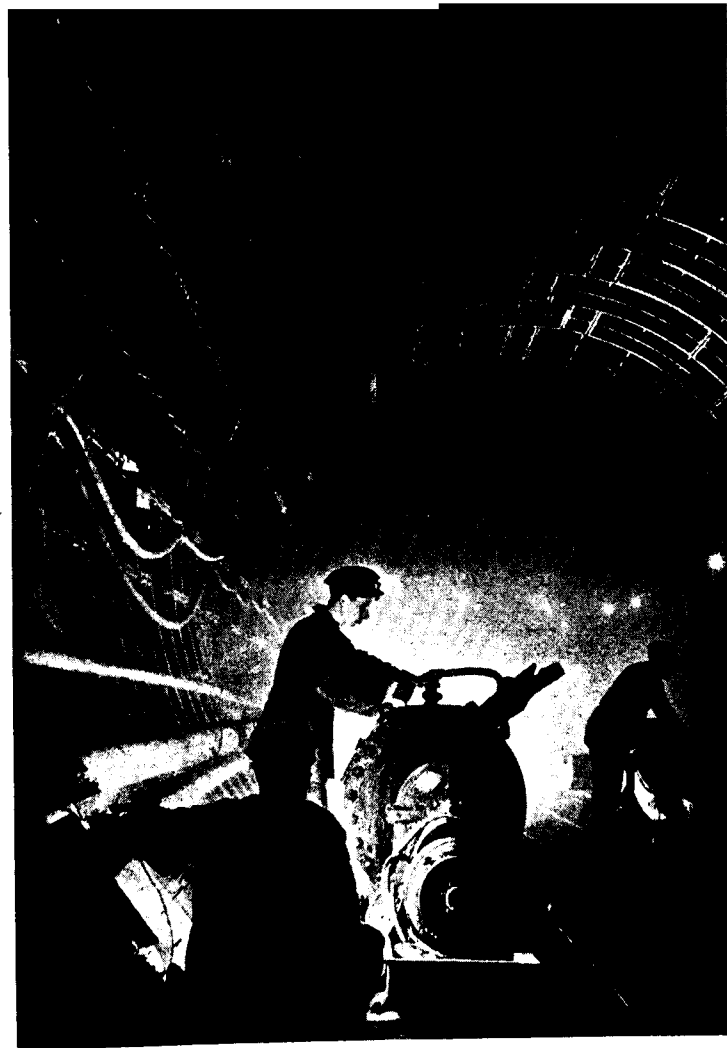
17. Tunnel on Don Trunk Canal. Fed from the Tsimlyanskaya reservoir, the canal will supply water for the irrigation of 1,850,000 acres, and will provide water for livestock over a wider area. It will be in four parallel tunnels, each 6 km. long, beneath the Don-Sal watershed.
