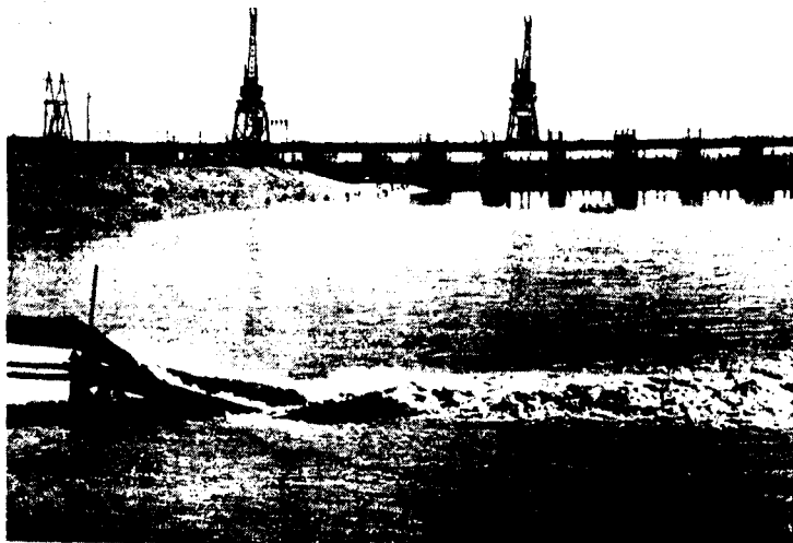
3. Tsimlyanskaya site (River Don): filling the spillway hollow. After river-level had been reached, and free access provided from river to spillway, blocking of the natural channel was completed: large quantities of concrete were dumped quickly in the final stages.
