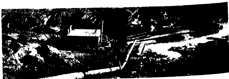
10. Volga-Don navigation canal: suction dredge at work (December 1951).
