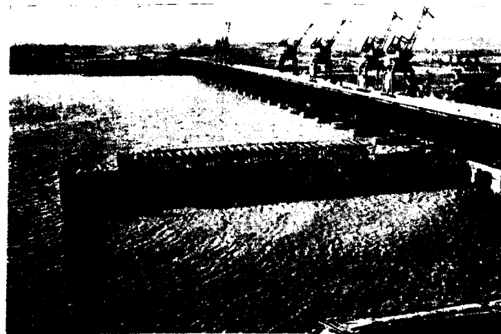
5. Tsimlyanskaya site (River Don): as Inset 4 (above), but after filling to river level. The extent of backing-up which will be effected is indicated by the excess-height of the spillway dam. The appearance is of 'dead' water at this stage.
