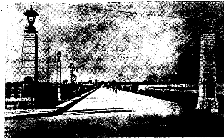
The Road Bridge on the Nangal Dam
