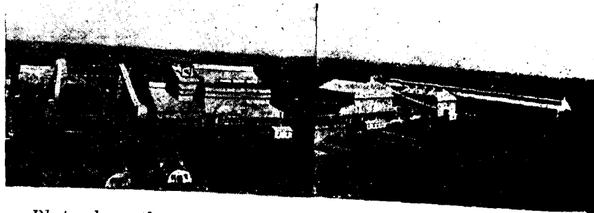
Photo shows the Sulphate Plant of the Factory. In the background is the 600 ft. long reinforced Concrete Silo capable of storing 90,000 tons of Ammonium Sulphate.
