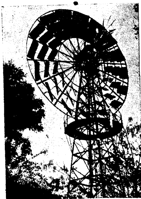
Stand by windmill for pumping well water. Locomotive workshops, Ajmer.
