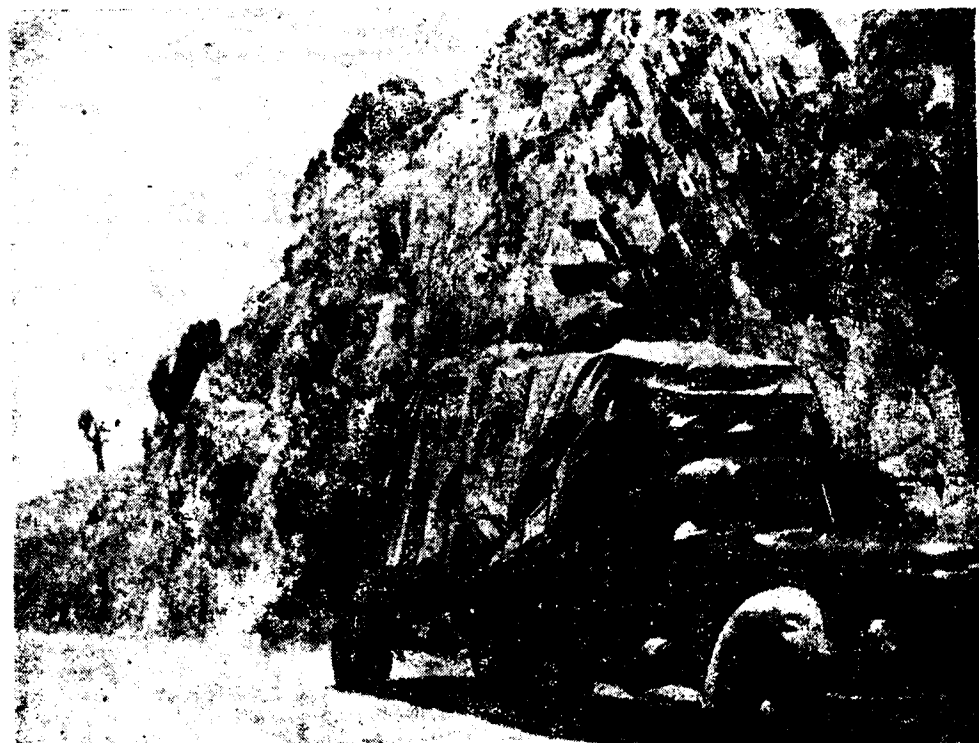
Heavy work in Rough Country
