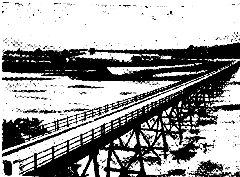
Jandola Road Bridge, North West Frontier Province, 38 R.S. Joist Spans, 36-feet, on Screw Pile Piers.
