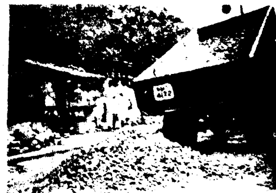
Figure 2. Coarse aggregate being dumped on the subgrade.
