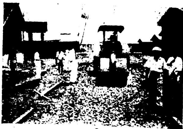
Figure 4. Rolling coarse aggregate.
