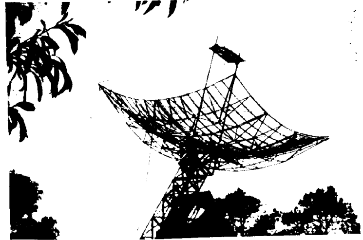
25. A modern radio-telescope in use near Sydney, Australia. It is fitted with a parabolic aerial reflector of dimensions 16 feet by 18 feet and can be used at wavelengths of 1\frac{1}{2} metres, 50 centimetres or 25 centimetres.
