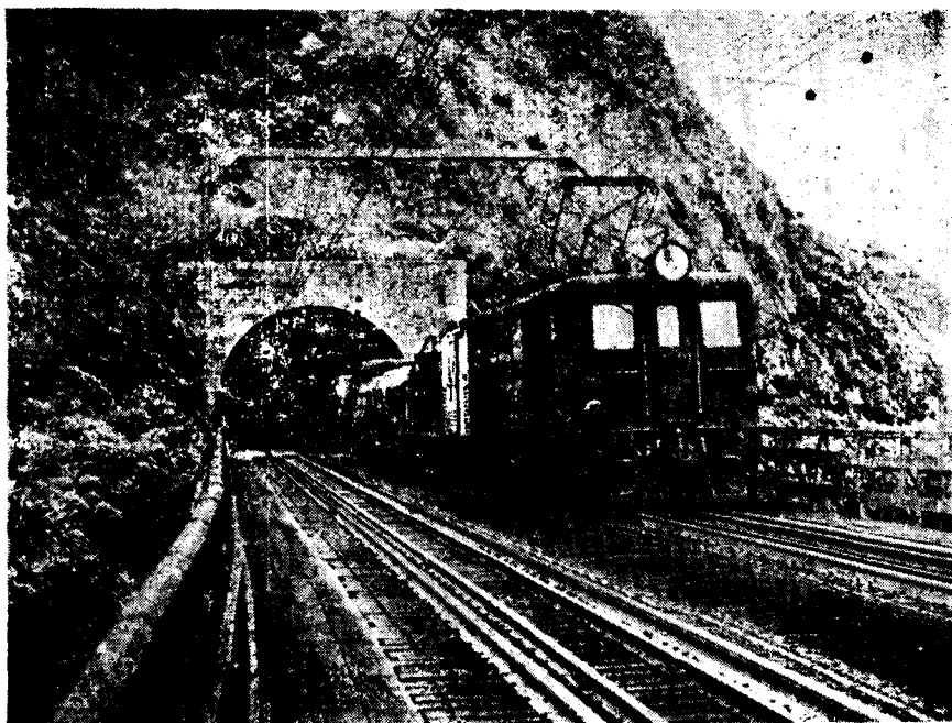
Class "Ed" electric locomotive entering Wellington on the present main line
