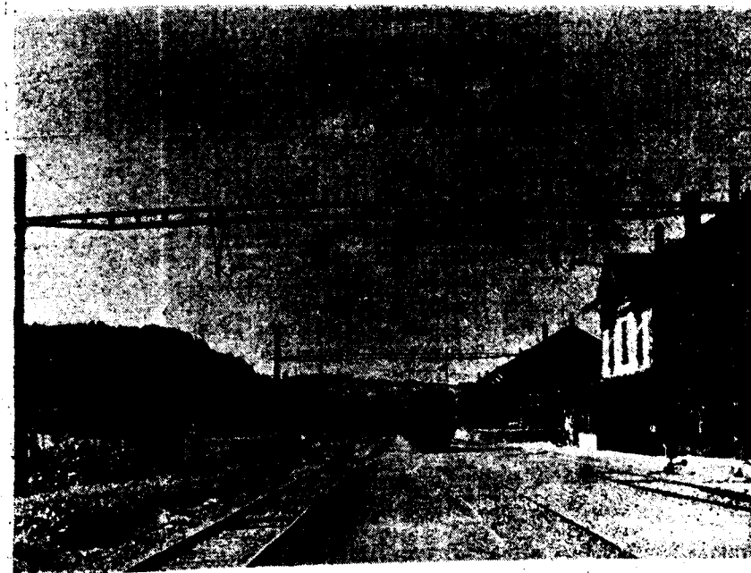
15 kV S. B. B.—contact line (station)
