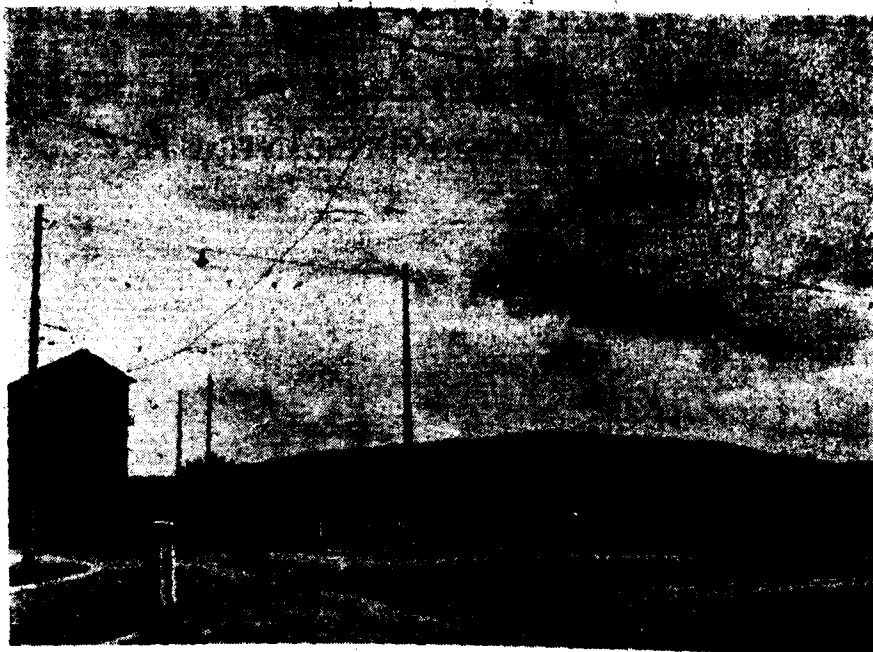
Full elastic suspension of the contact line for Tramway (pantograph) in curves
