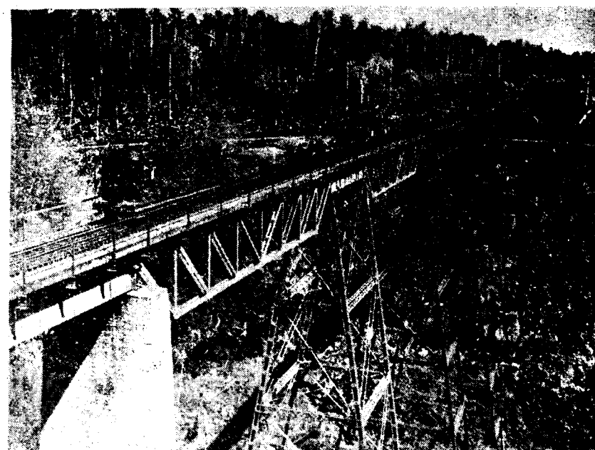
Goods train crossing the Makotote viaduct, Wellington Auckland Railway. The bridge is 260 feet high and 860 feet long.
