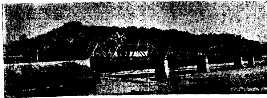
The Tista Bridge. Central Span of 250 ft. Clear with two spans of 150 ft. on each side.
