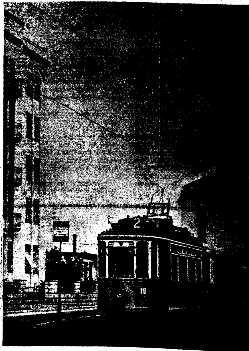
Full elastic suspension of the contact line for Tramway (pantograph) on straight line
