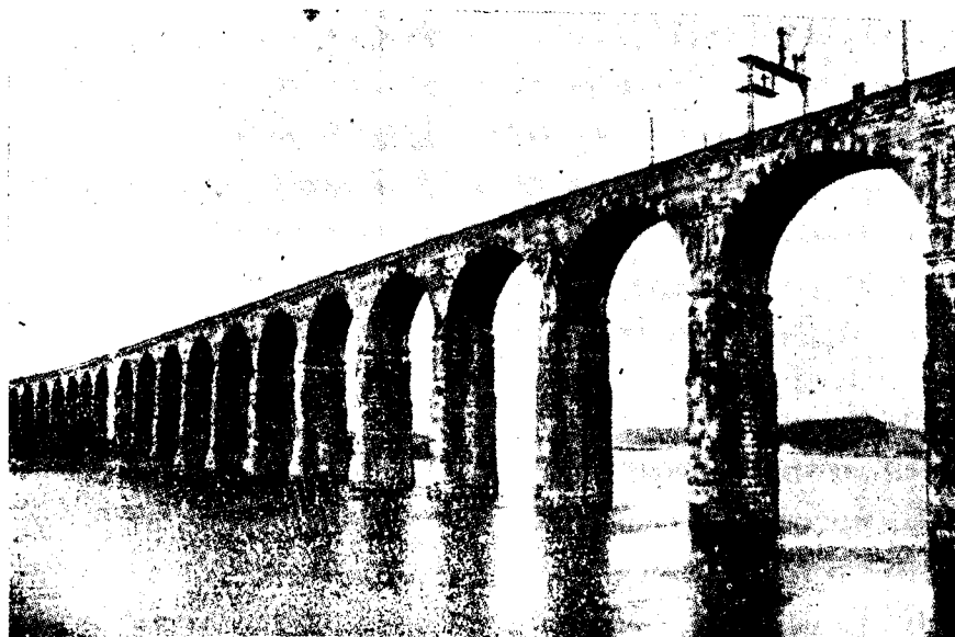
The Royal Border Bridge carrying the British Railways East Coast line across the Tweed at Berwick opened by Queen Victoria on August 19, 1850. It is now over hundred years old.
