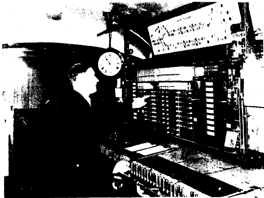
View inside control cabin at Mount Pleasant. The slides by the switchman's right hand control the entrance and dispatch of the miniature trains. The push buttons above work platform signs for the direction of the loading and unloading staff.
