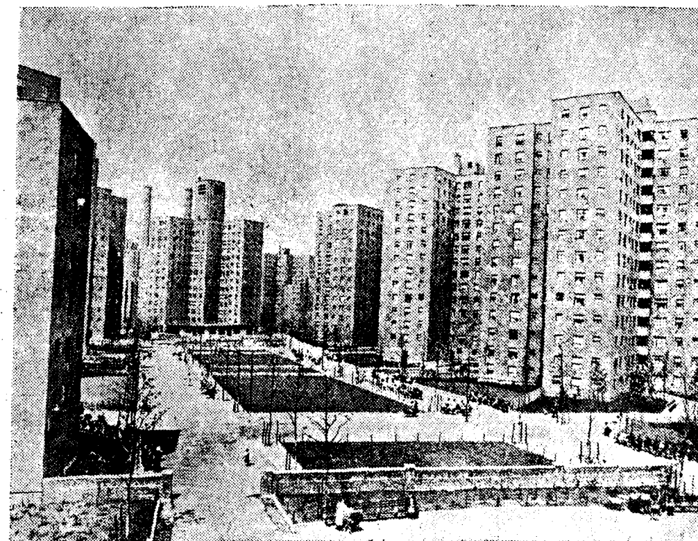
These stately apartment houses with park and play space about them are replacing slum conditions in many American cities as part of the nation-wide, low-cost housing program sponsored by the Federal Government.
