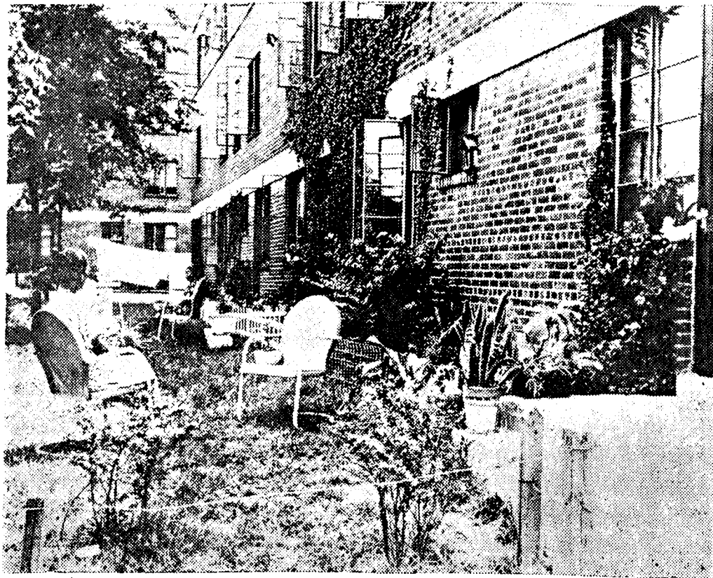
Light, air, privacy, and individuality are shown in these simple but attractive dwellings which are springing up in many American cities as part of the national low-cost housing programs.
