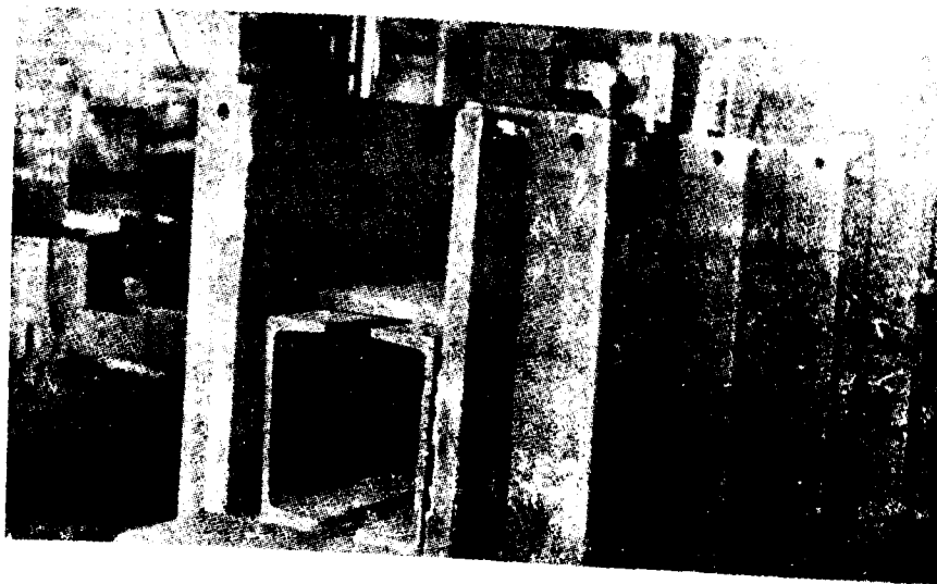
SHOP WELDING a heavy truss member (20 X 14-in. flanges and 10 X 4-in. web) for a 192-ft simple span. Plates are tack-welded in an assembly jig.
