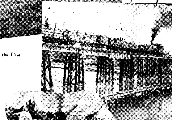
One of the many pile bridges used to expedite construction
