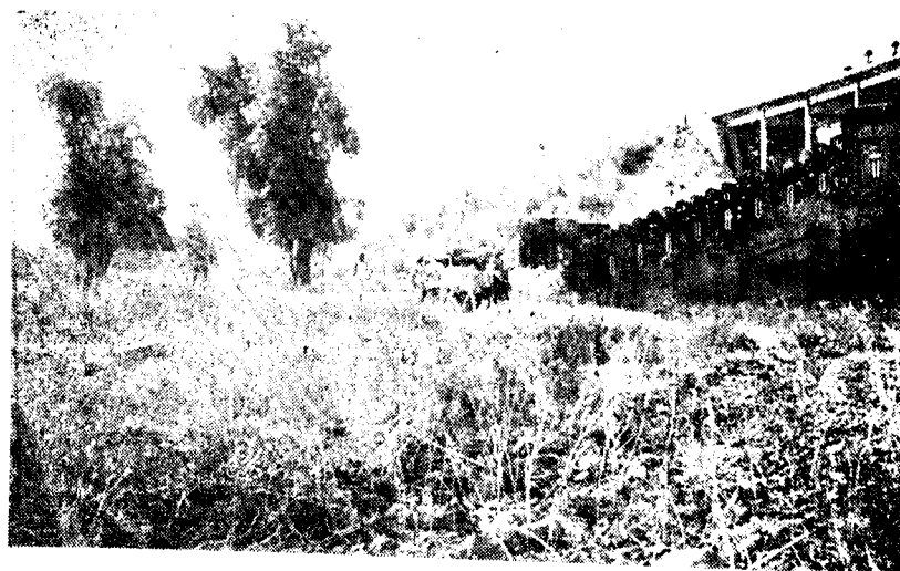
Photograph 1. A View of the Moghalsarai Side Approach.
