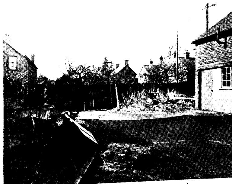
General view of inside the yard, including the storehouse
