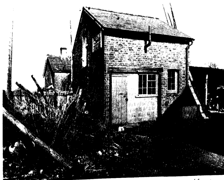
Close view of storehouse
