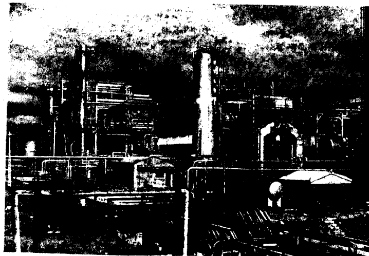
2. A view of the Hydrocarbon Fractionation Unit and on the right the Cracking Plant.
