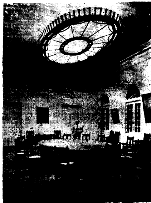
Probably the largest single Fluorescent Lighting unit in India. It is installed in the Council Room of the Indian Institute of Science, Bangalore.
