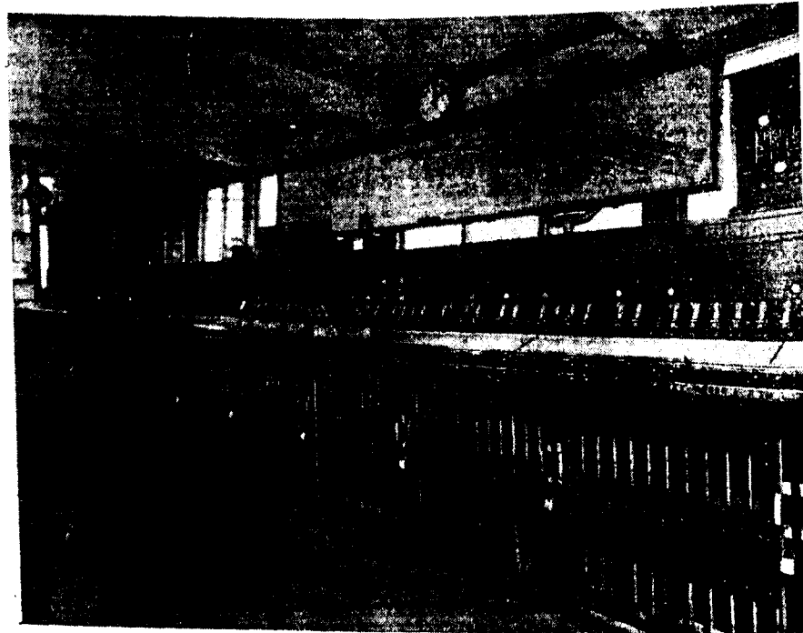
140 Lever all electric interlocking frame at Fenchurch Street, London & North Eastern Railway.
