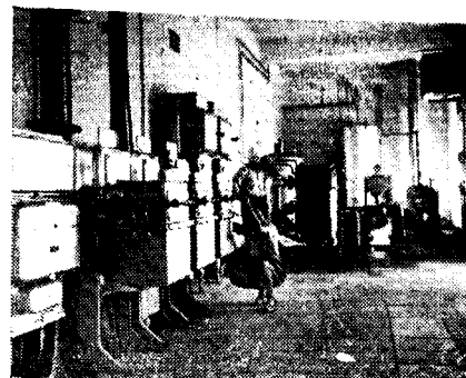
Compressor, Switch-Gear & Boiler Room
