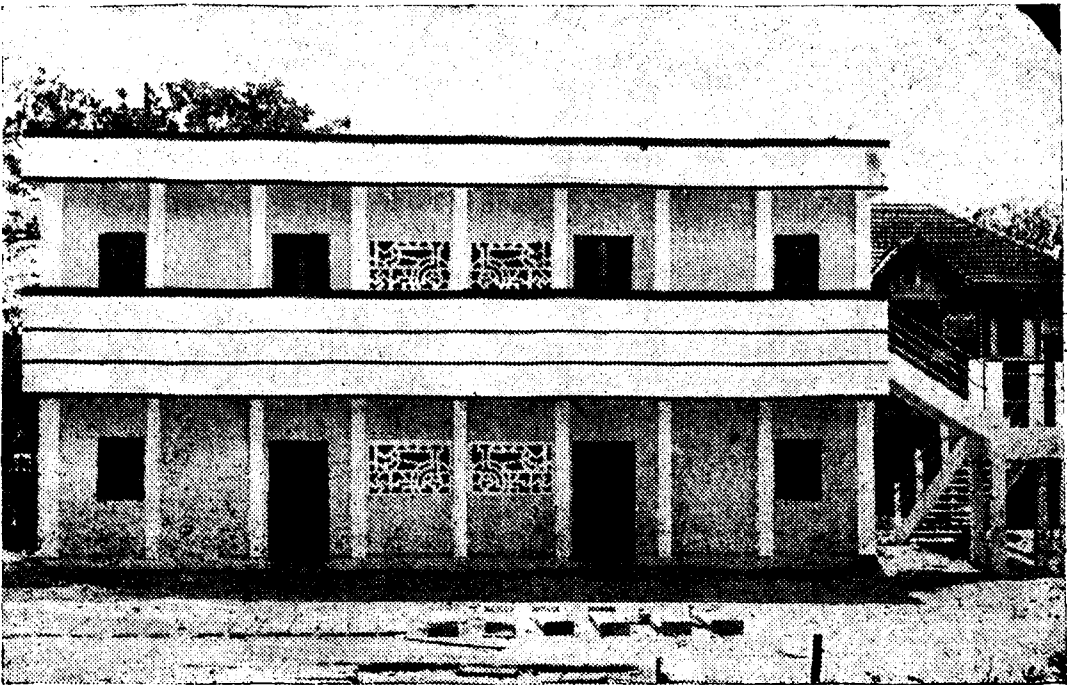
Fig. ix. Prefabricated, single wall, double floor, flat roof GUNITE HOUSE at Vile Parle, Bombay.
