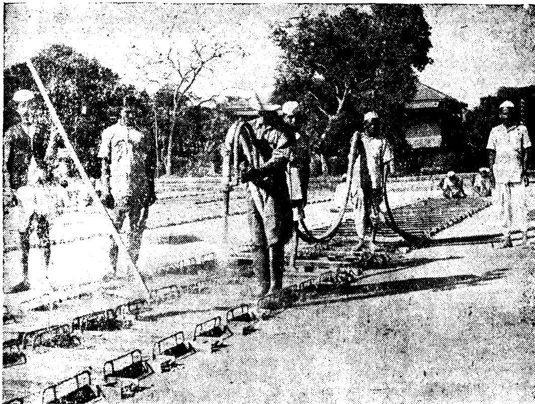
Fig. vii. Casting of slabs by guiding at Bulsar Bridge Depot
