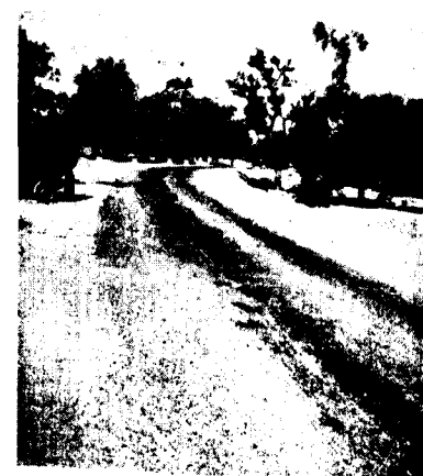
Photo 3 Showing second coat painted surface in mile 23 ; the portion in the foreground is with normal grit and in the back-ground with bitumen coated chips
