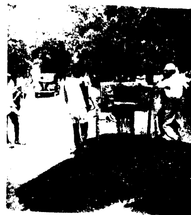
Photo 1 Showing preparation of precoated chips by hand-drum mixer
