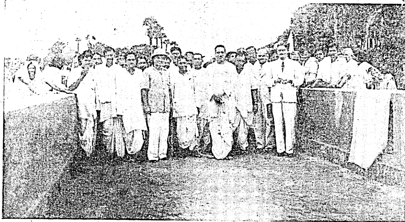
The Hon'ble Premier, Sri P. S. Kumaraswamy Raja, and Sri K. Chandramouli, Minister for Local Administration, at the opening of a bridge at Pittalavaripalem, Guntur District.
