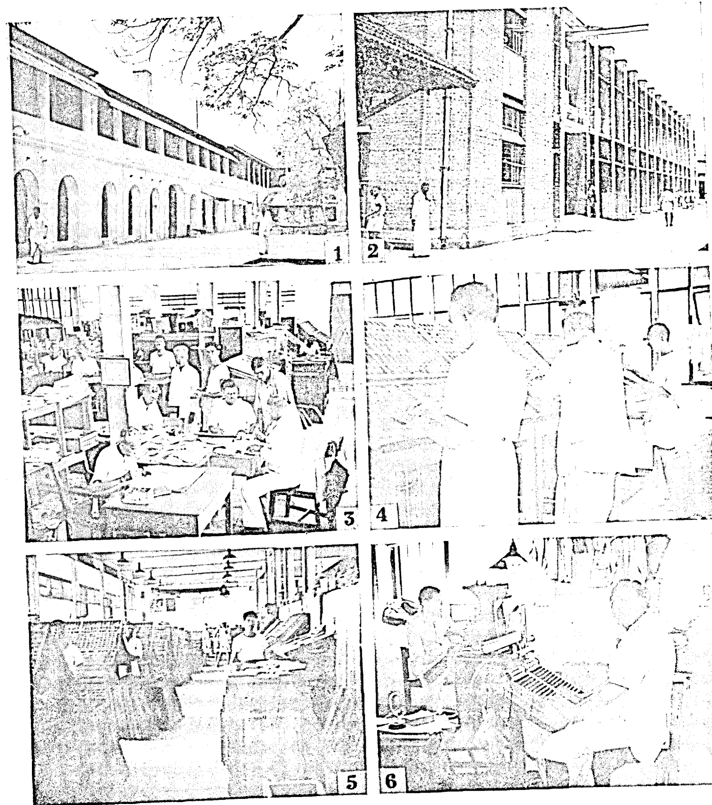
(1) Government Press Building Administrative Section. (2) Government Press Manufacturing Department. (3) I. & P. Composing Department (War Section). (4) Setting up 'Information' work in Indian languages. (5) Work in progress. (6) Monotype machines.
