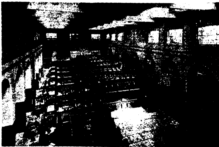
Plate 30. The Pumping Station at Mogden. The vertical scale on the left registers the depth in the suction sump of sewage to be pumped to the upper level.
