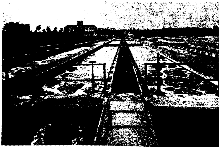
Plate 31. Aeration channels showing mixture of sewage and activated sludge being agitated by compressed air. (Both photographs by courtesy of the Middlesex County Council).
