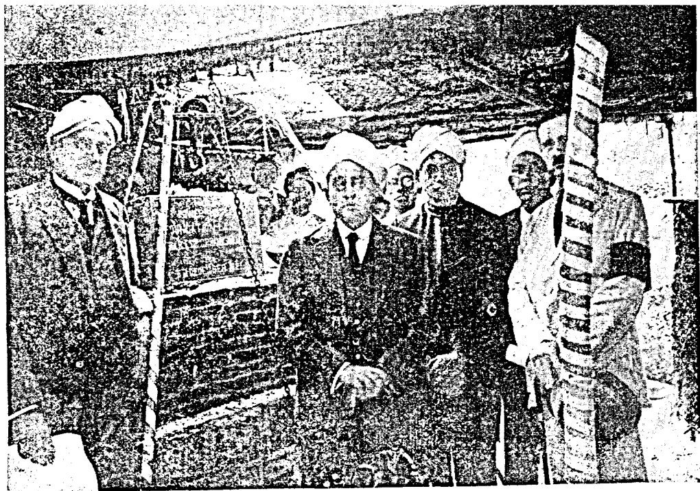
SIR C. P. RAMASWAMI AIYER laying the foundation stone
