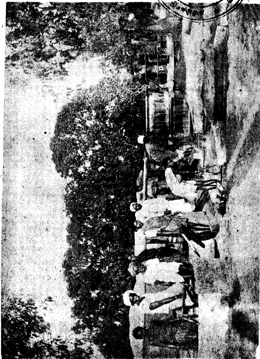
Look ! How sand is washed for slow sand filters ! Why then blame them for yielding poor results ?
