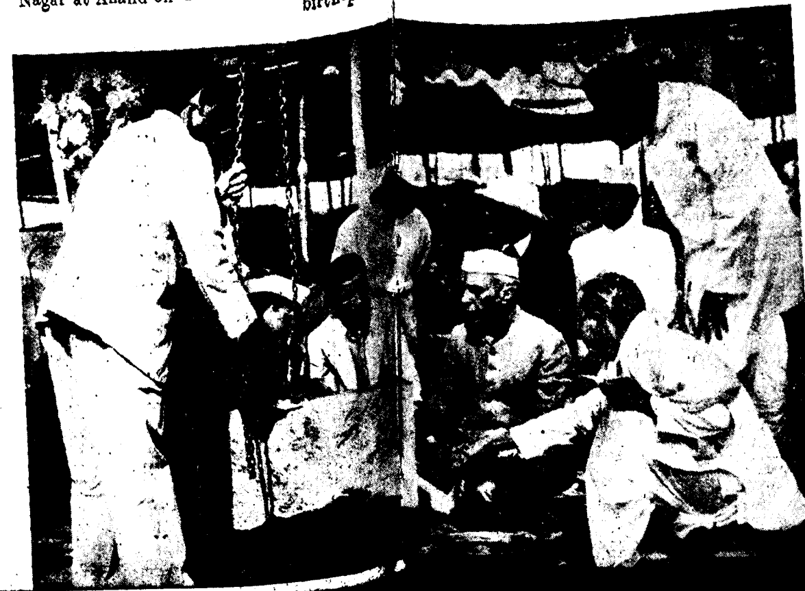
Pandit Nehru unveiled a bust of Sardar Vallabhbhai Patel, the Deputy Prime Minister, at Godhra on Feb. 13. (Below) The Prime Minister laying the foundation stone of Vallabh Nagar at Anand on Feb. 13. The new township is on the border of Karamsad village, the birth-place of Sardar Patel
