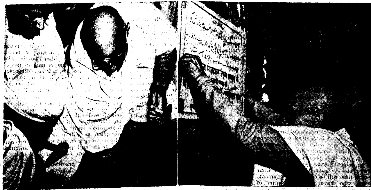
Shri C. Rajagopalachari laying the foundation stone of the memorial at Victoria Park, Banaras, the place where the last remains of Mahatma Gandhi are kept for public view. (Right) The Governor-General laying the foundation stone of the Mazharul-Ulum Orphanage at Banaras on December 1
