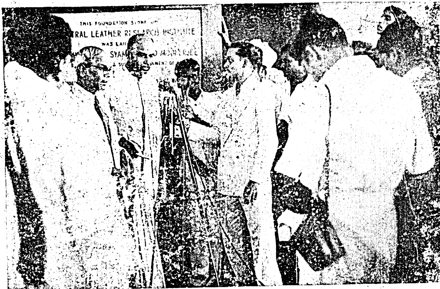
Honourable Sri S. F. Matherjee, Minister for Industries, Dominion Government, laying the foundation stone of the Central Leather Research Institute at Guindy, Madras
