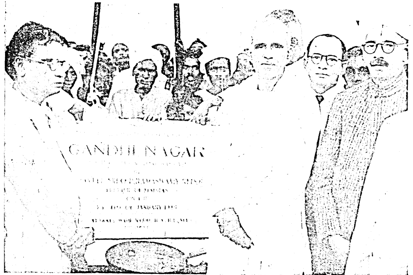
Another milestone in the solution of the Housing problem in Madras—a triumph of Co-operation. Here is seen the Hon'ble Premier of Madras laying the foundations of Gandhi Nagar a township sponsored by the Madras Co-operative House Construction Society
