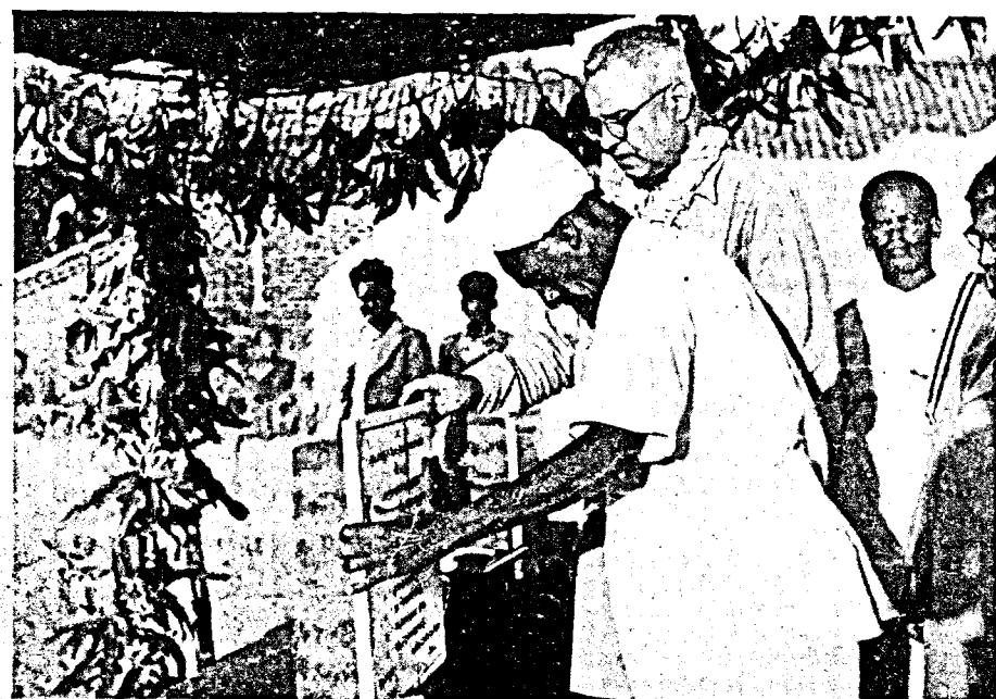
The Commissioner of Prohibition laying the foundation stone of a godown-cum-community centre in North Arcot district. These centres bid fair to become the hub of village life in the future
