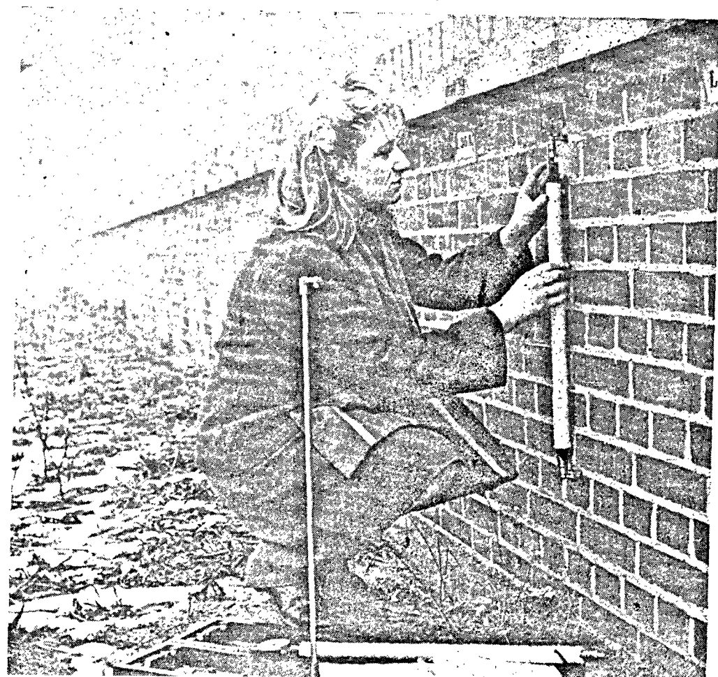
A careful check is maintained on changes occurring in brick walls and similar structures. Steel balls built into the wall are used to provide very accurate measuring points for the determination of shrinkage.
