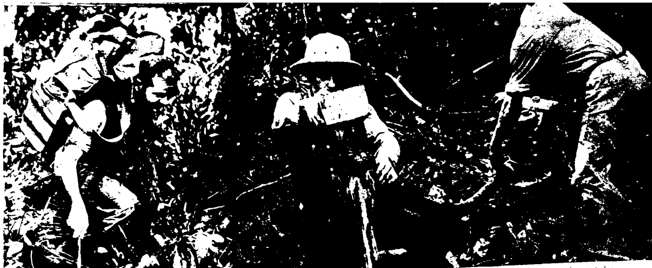
Plate 5. Priming the water-pump by pouring water into the intake head, which will then be dropped into the slush pit. The pump, under the hands of the man on the right, drives water through the line in the background to the drill (plate 4).
