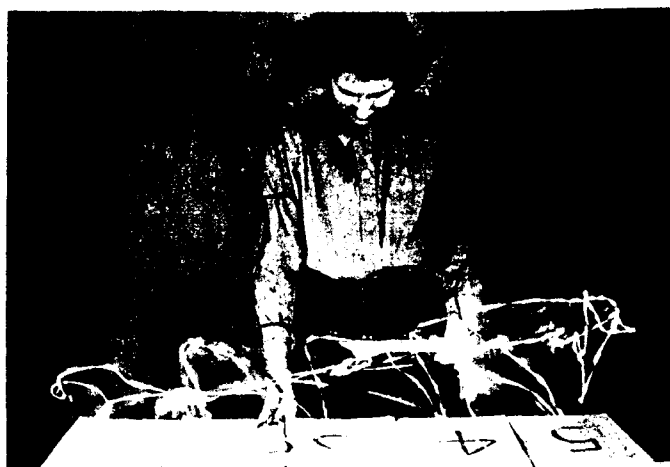
Plates 42 and 43. Micromotion study of the Collation of Documents. (See also page 107). The girl had small lamps strapped to her wrists so that her hand movements in sorting papers could be recorded by long exposure on one plate. Notice how much more economical of effort is the arrangement in the lower picture.
