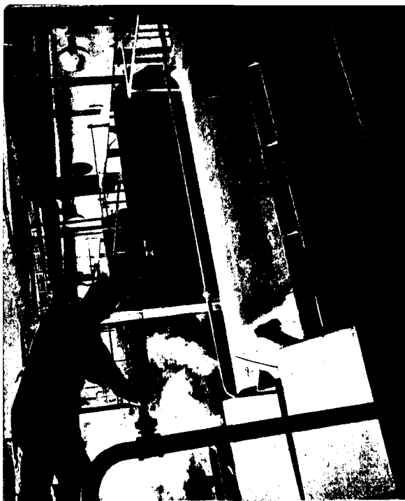
15. The new way: One of a number of 25-foot 5,000 gallon fermenters or vats in which the growing mould feeds upon its nutrient medium.
