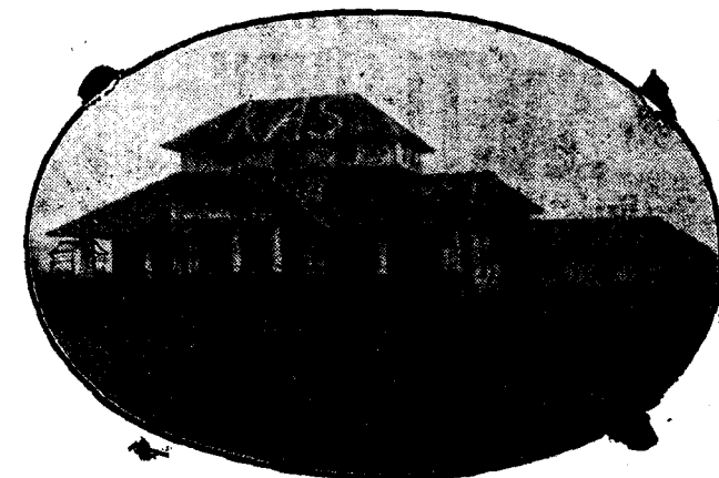
Front view of the Main Hospital at Shoranur.
