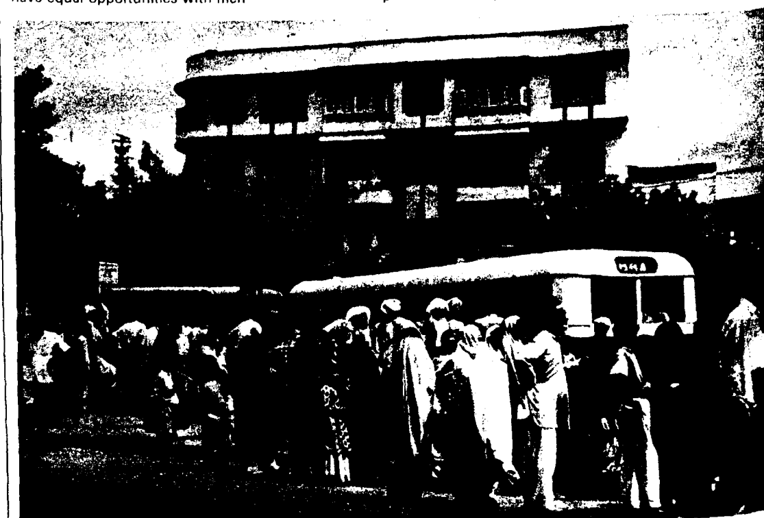
A typical roadside scene with burqa-clad women waiting at a bus stop
