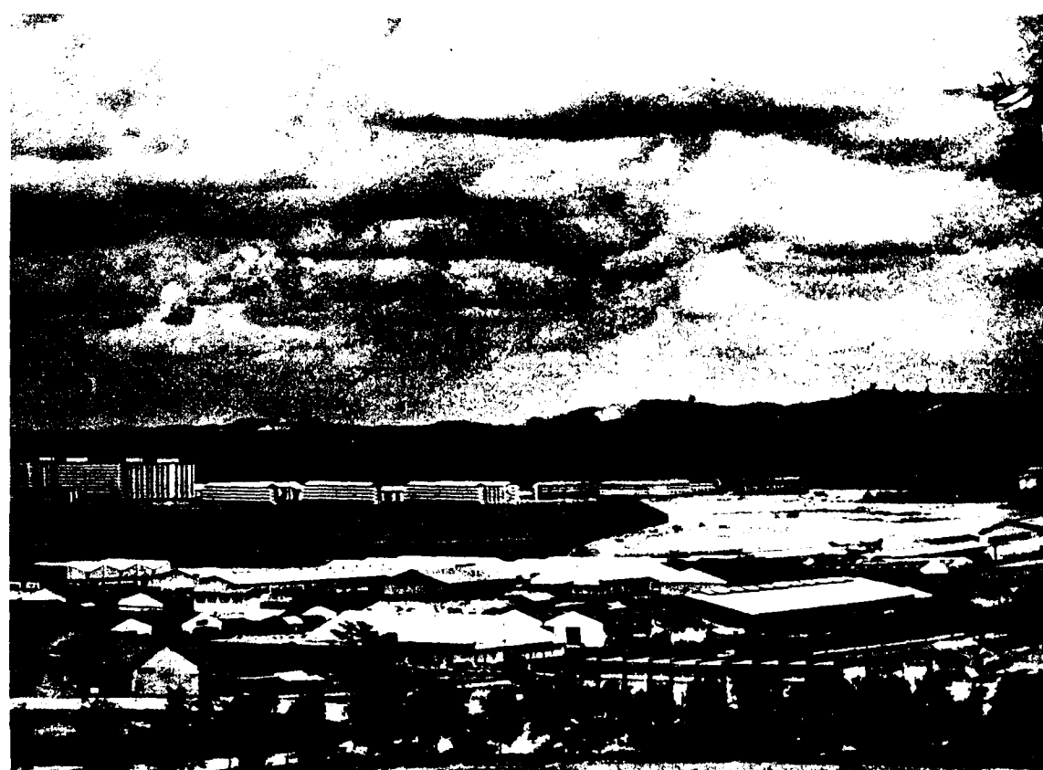
A section of Jurong Industrial Estate which only five years ago was a mass of mangrove swamps and prawn ponds. Today it is the admiration of south-east Asia. To service the estate 18 miles of main roads have been built, a nine-mile railway laid, and electric sub-stations, reservoir and an industrial water plant constructed
