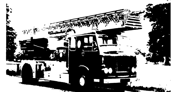
This vehicle has been specially built in Britain by Dennis Bros. Ltd., Guildford, for the fire-fighting department of the Municipal Council, Colombo. The ladder can extend, elevate and slew at the same time.
