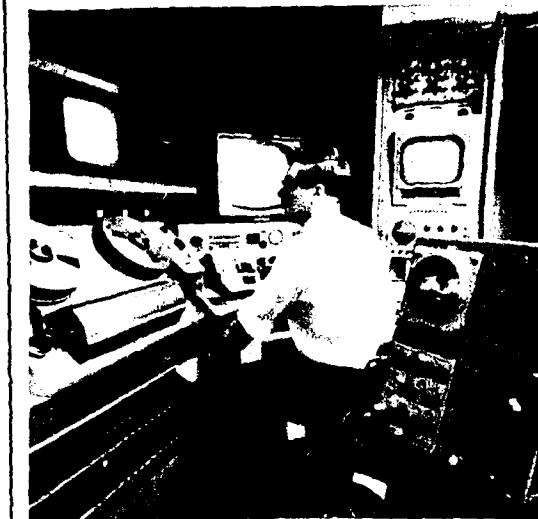
A great many programmes have to be pre-recorded for one reason or another; plays, for instance, can only be recorded when all the actors are available. This is done on a video tape recorder on which both the picture and sound can be preserved for further use
