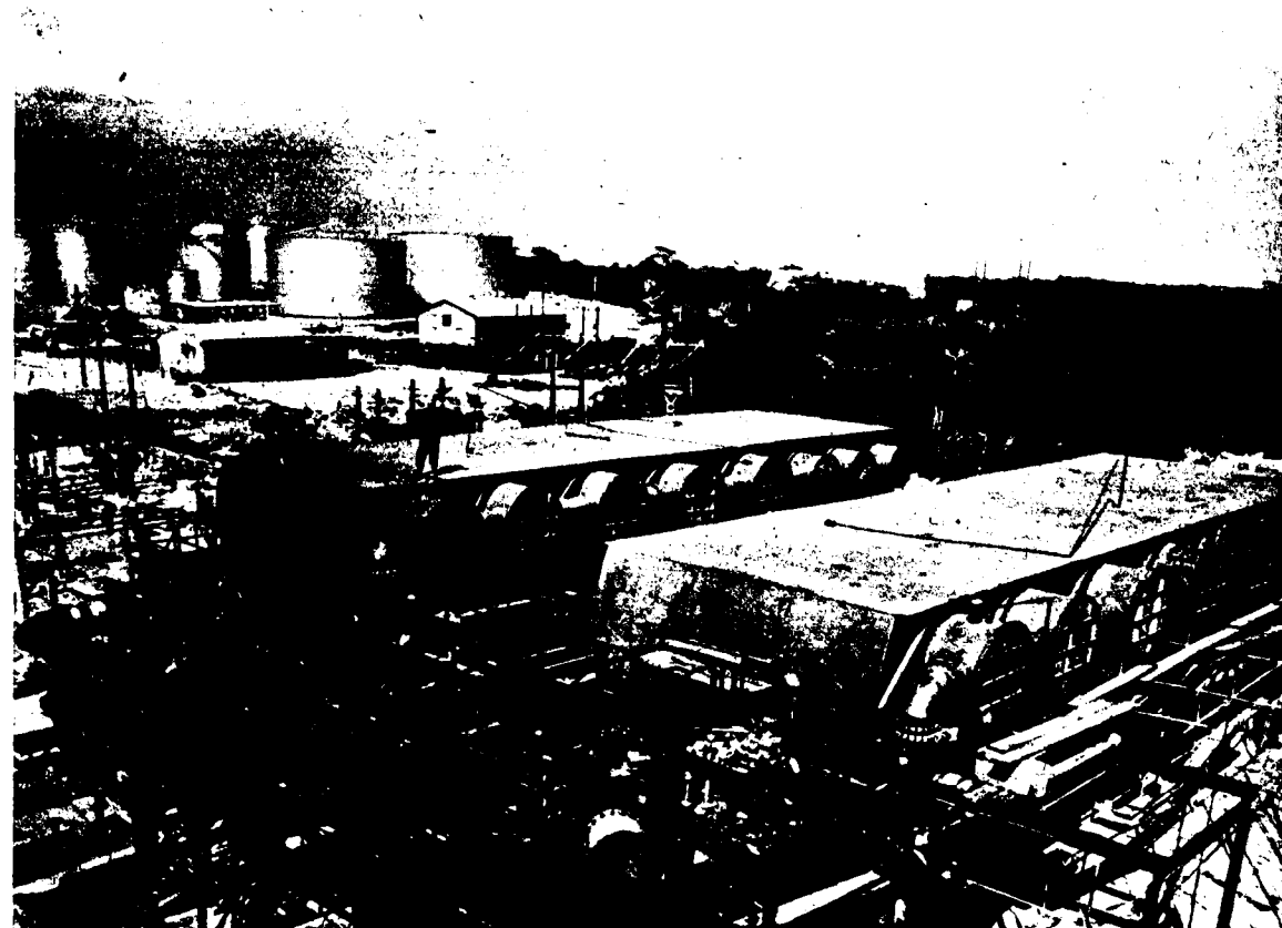
Two British-designed evaporator plants in the Bahamas, each producing 600,000 gallons per day
