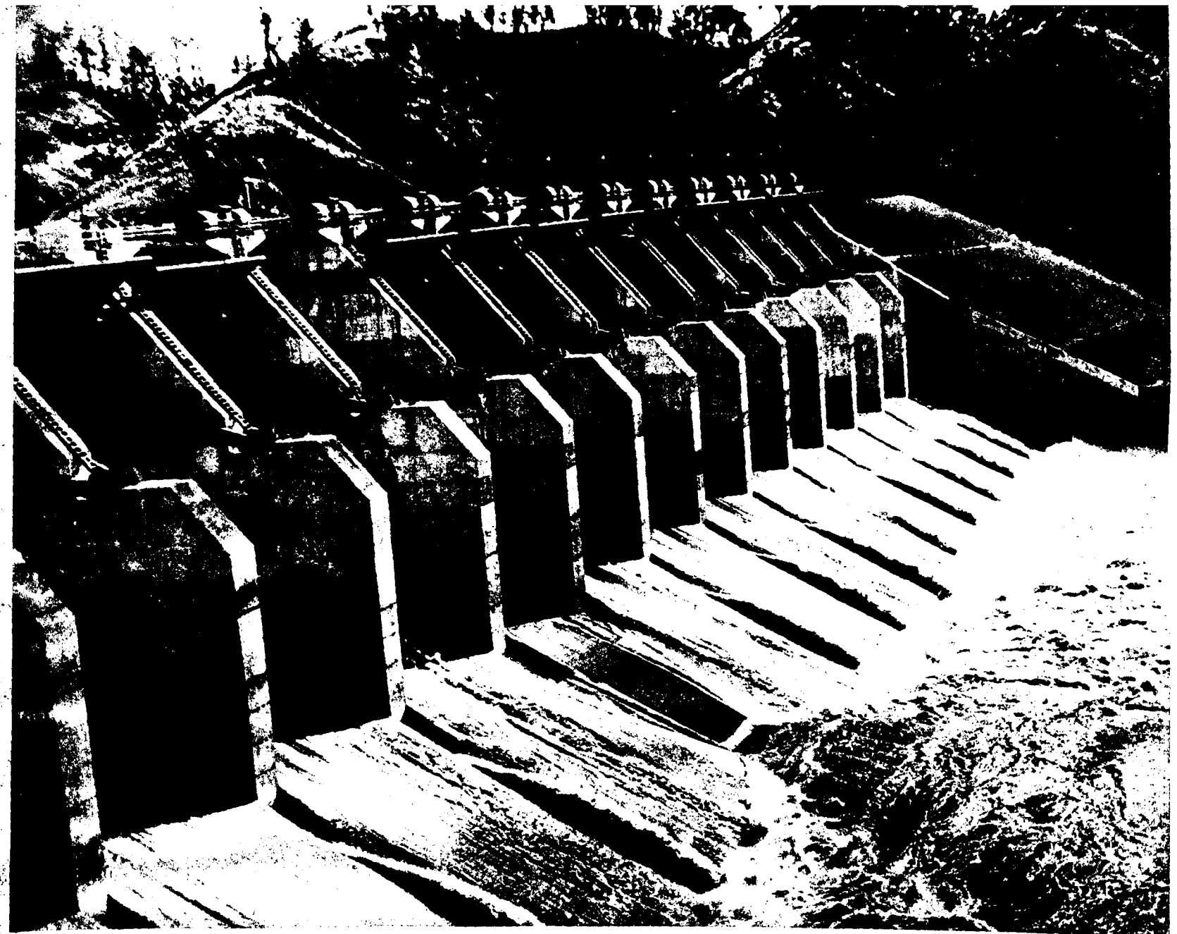
A spillway of the Karnafuli hydro-electric project at Kaptai, first and biggest hydel power project in East Pakistan
