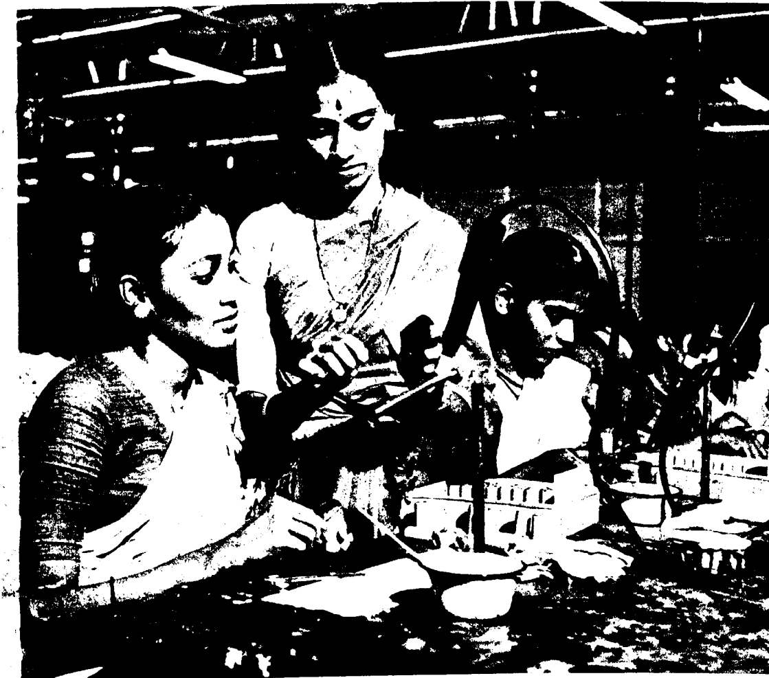
The English Electric Company of India Limited, employs about 1,000 people in its Madras factory. It began full operation in 1961 and is one of the most up-to-date factories in India—designed by Prynne, Abbot and Davies of Britain. This picture shows a female operator being given tuition in the small fuse assembly department
