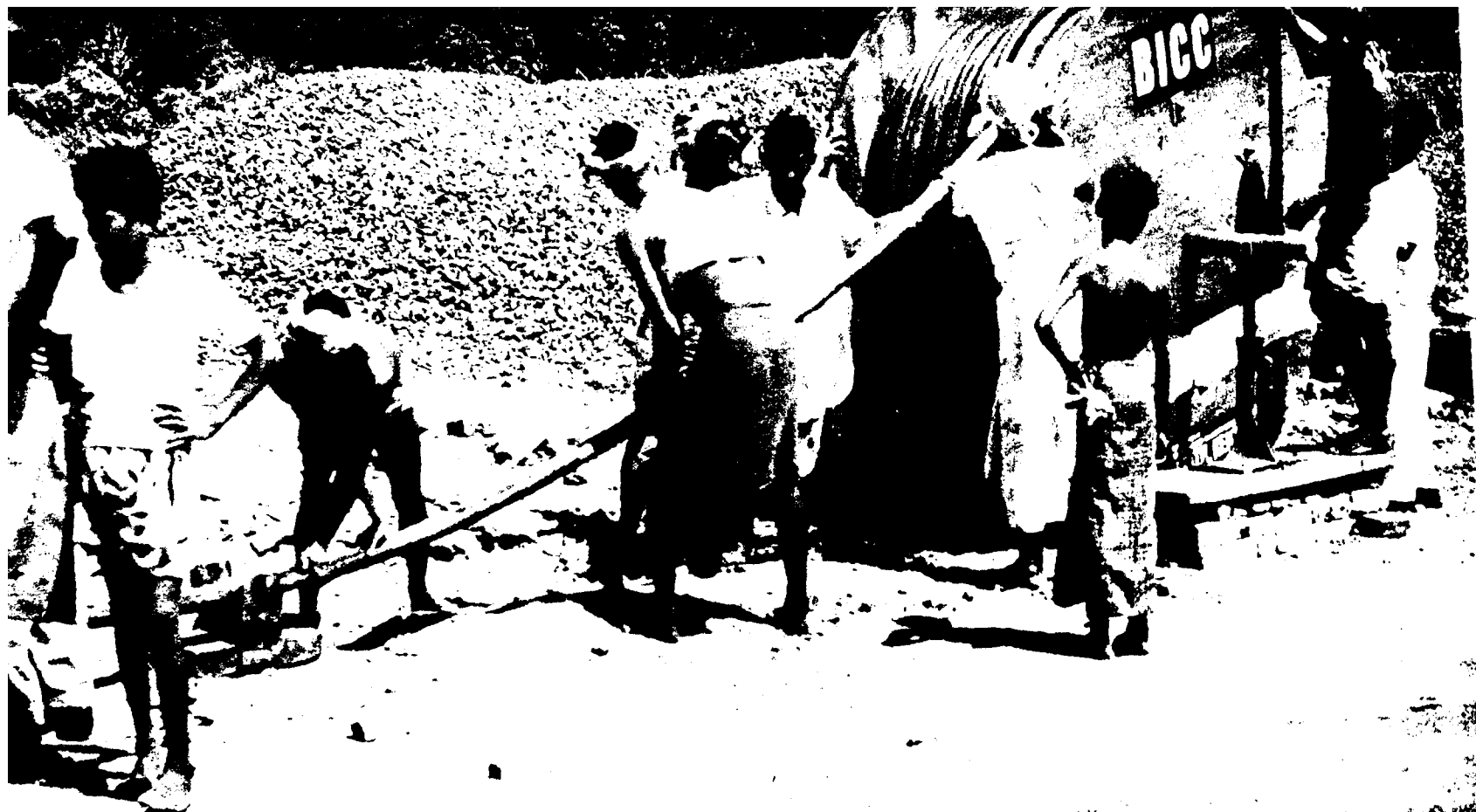
Pulling the self-supporting aerial power cable off its drum on the 11 kV cable route between Dhanmandi thermal power station at Dacca and the new East Pakistan radio transmitter, Savar
