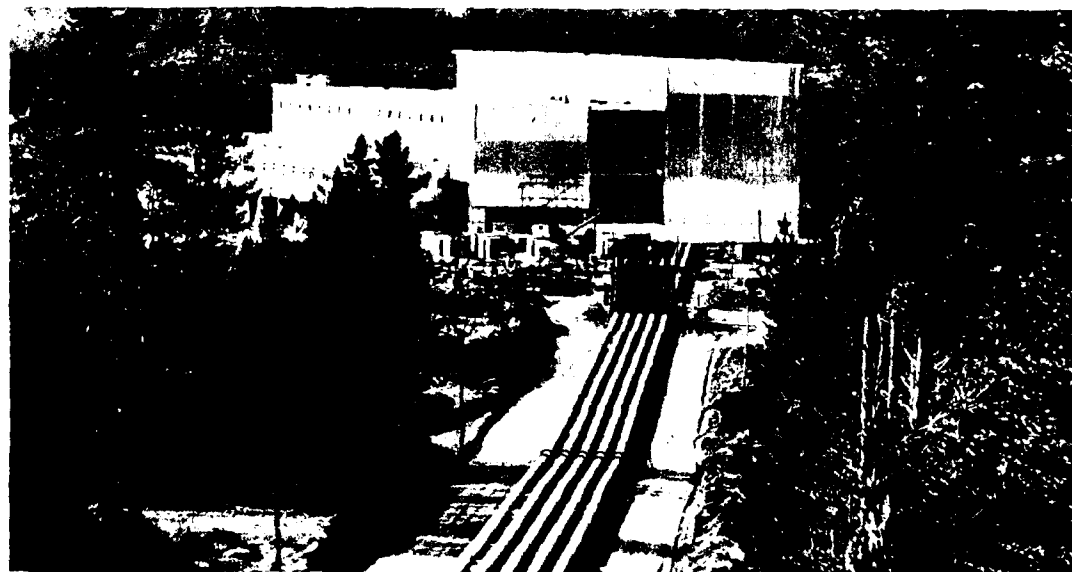
Opposite page: Wairakei, New Zealand, where man has tapped subterranean power and the earth breathes boiling water and steam. Left: These men preparing to "blow" a new geothermal bore are constructing a concrete casing which will act as a silencer when pent up steam roars into the atmosphere. Below: A power house at Wairakei, nearing completion. It measures 200 ft. by 200 ft. by 75 ft. high, and is finished in aluminium cladding and glass. Electric power from Wairakei is the cheapest in New Zealand.
