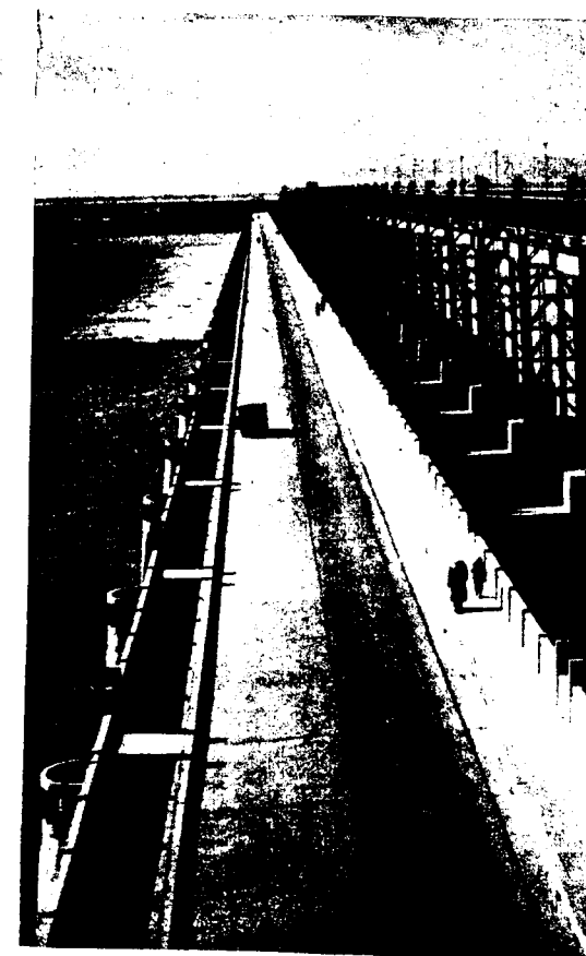
The Taunsa Barrage for irrigation of hitherto arid areas
