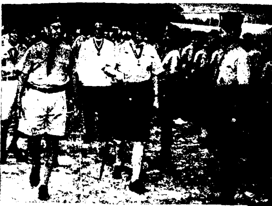
The Chief Scout of the Commonwealth, Sir Charles Maclean (centre), inspects Scouts at Jesselton prior to "turning the first sod" on the site of a new Scout headquarters in Sabah
