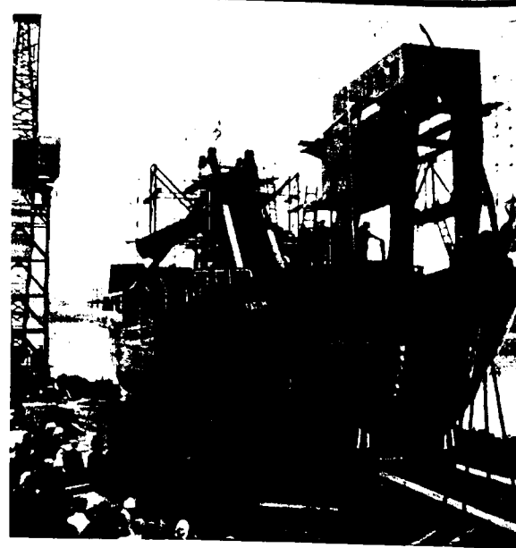
The "Fateh", first of two bucket dredgers specially built for Karachi Port Trust, starts on her journey down the slipway at Fleming & Ferguson's shipyard at Paisley in Scotland
