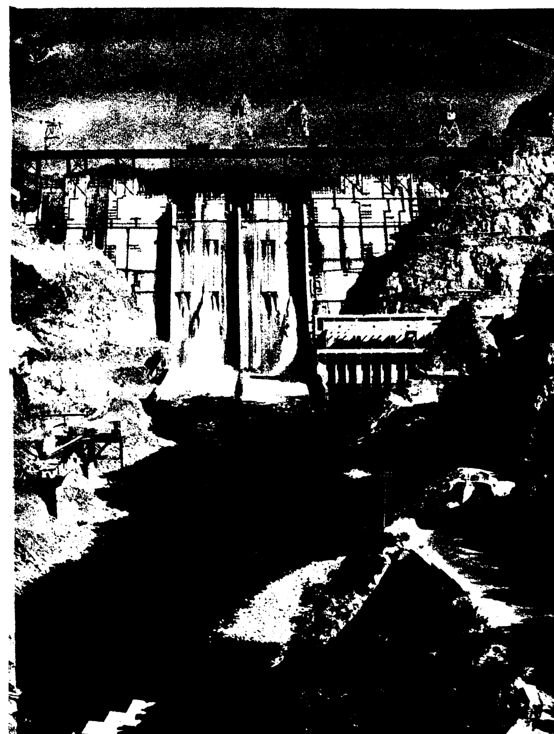
The Bhakra Dam : to lay the foundations, digging to a depth of 190 ft. below the river bed was necessary
