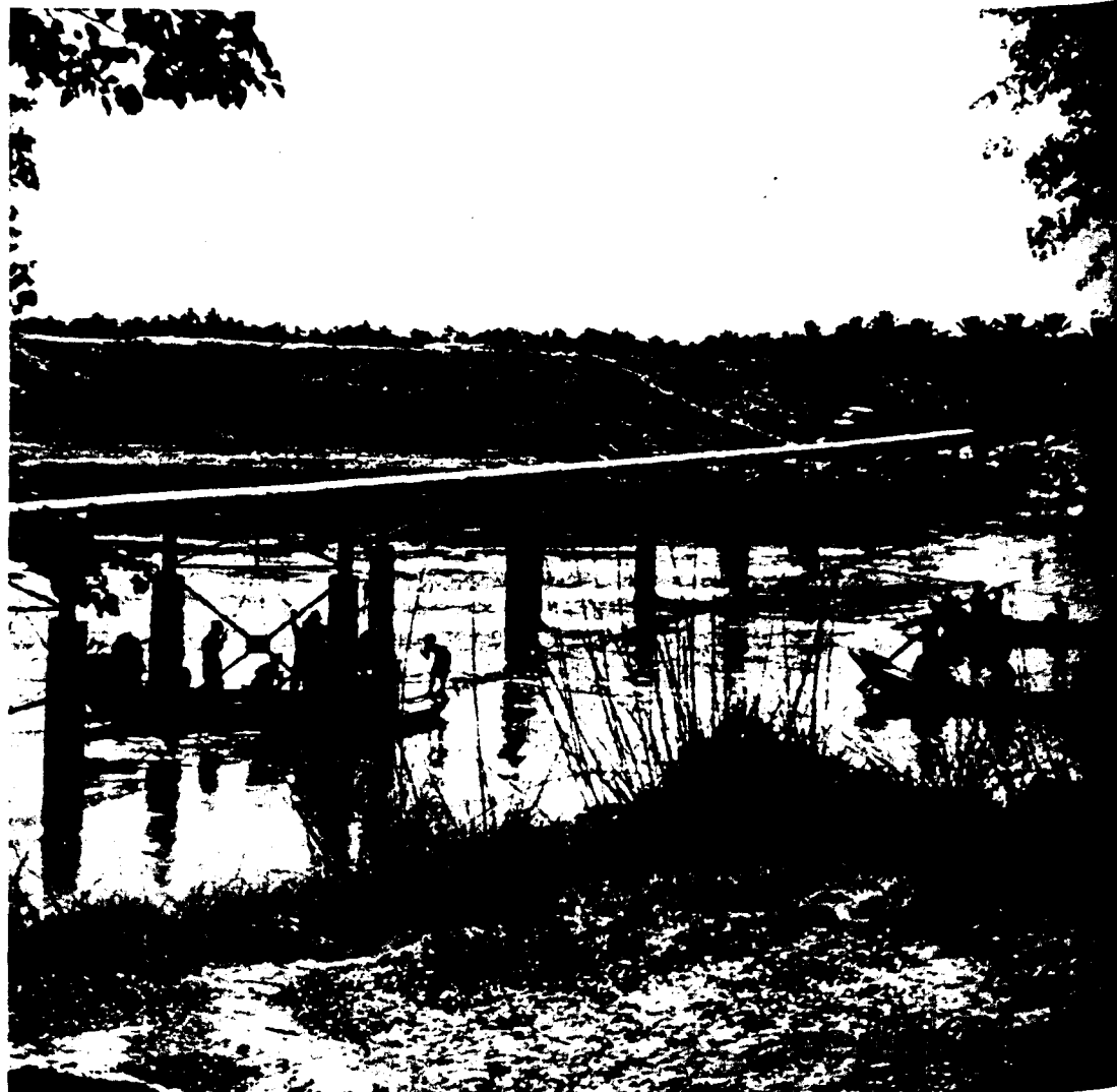
On its 347-mile journey from Sui to Karachi the gas transmission pipeline crosses every conceivable terrain. This picture shows one of the 54 canal crossings. Over 4,000 workers including 125 British and American worked round the clock to complete the pipeline in a record period of 168 days
