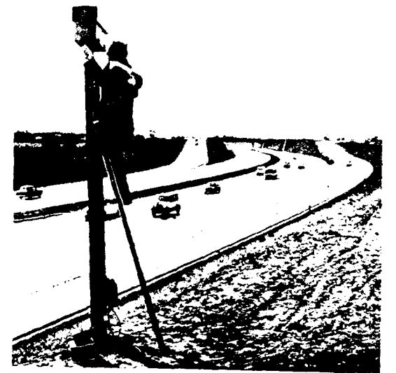
Adjusting a television camera beside a section of the M6 motorway, in the north of England. Pictures of traffic conditions are fed to monitor screens in a police control room.
