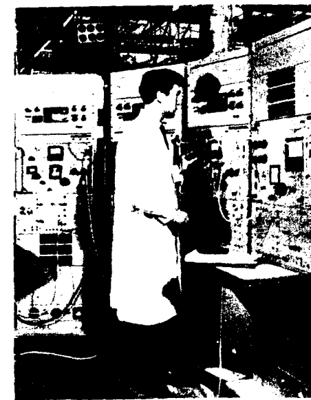
A.E.I. equipment that will form part of terminal stations at Hong Kong, Jesselton and Singapore for the first stage of SEACOM, the round-the-world Commonwealth telephone cable
