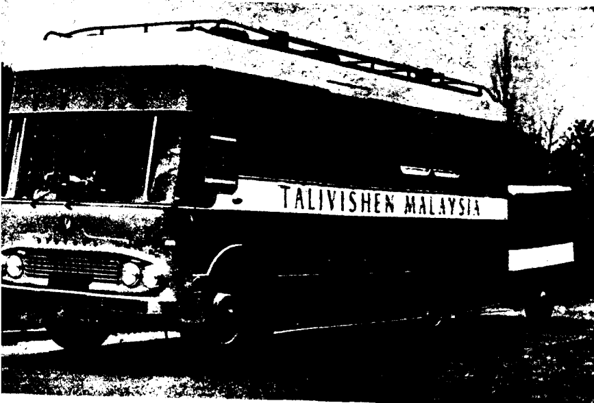
Round-the-clock shift work at Hayes, Middx., England, enabled EMI Electronics Ltd., to ship this outside broadcast vehicle to Kuala Lumpur in record time. The vehicle has three image orthicon cameras and associated equipment
