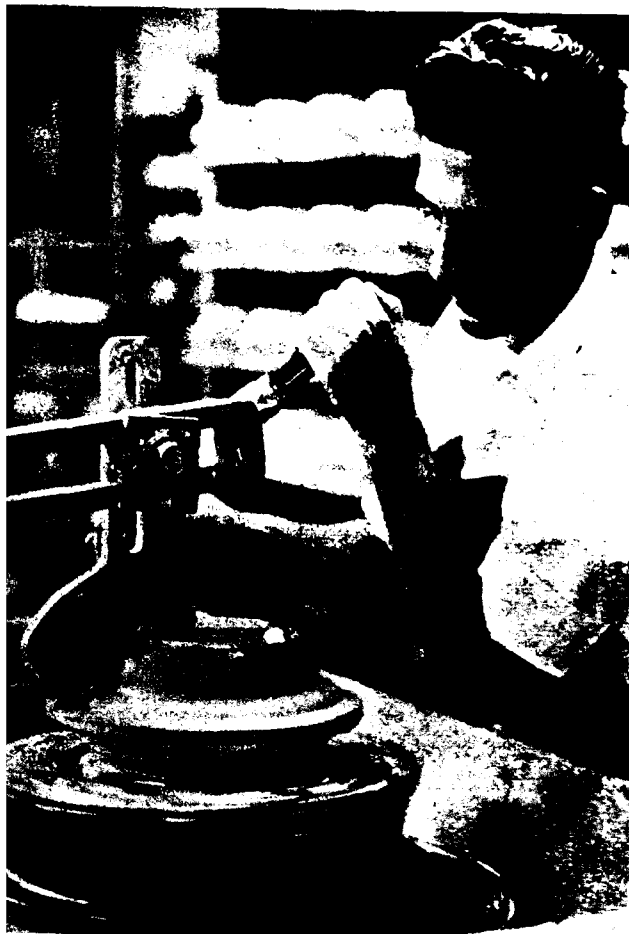
Clay is thrown on the spinning mould, shaped to the proper thickness by hand, and this profile tool used to shape the base
