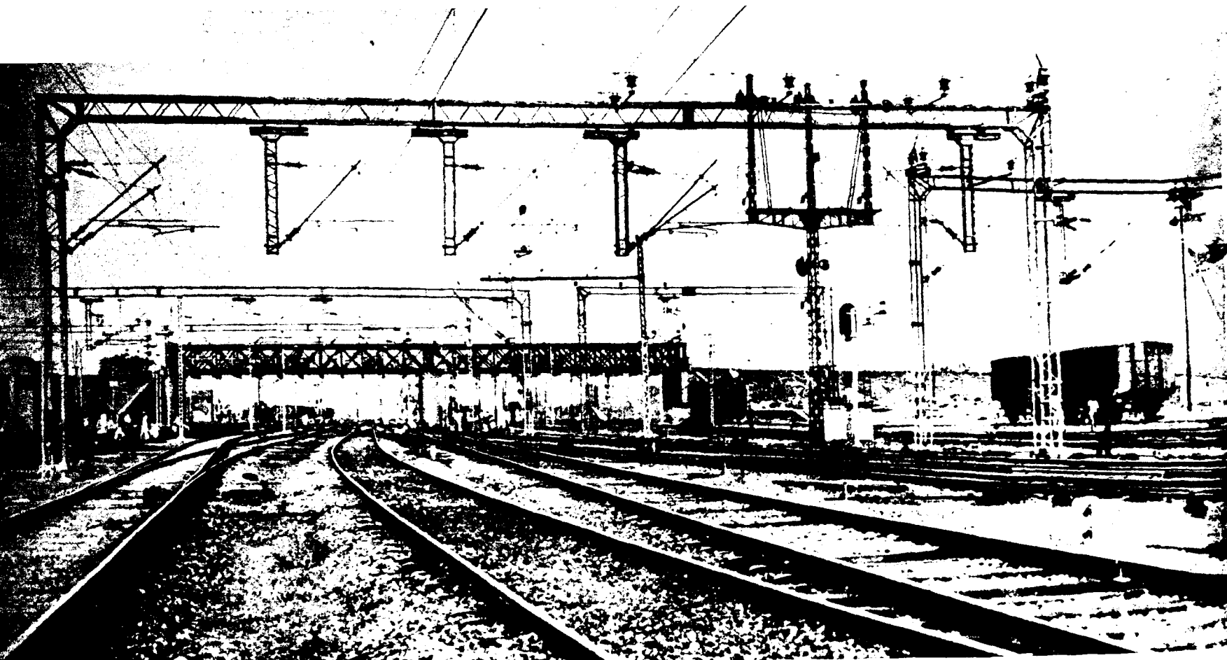
BICC overhead equipment for railway electrification at Moghalsarai on the Grand Trunk Line from Calcutta to Delhi. At Moghalsarai, BICC has completed electrification of one of the largest marshalling yards in Asia—155 miles of track. In all the BICC Group has received £8 million orders for work in connection with India's railway electrification programme.
