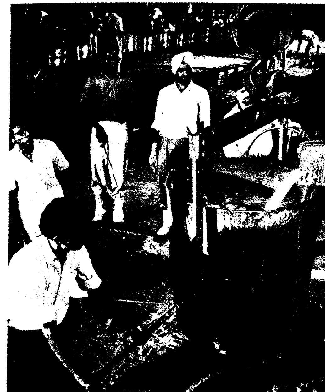
The foundry at the new factory for Heavy Electrical Apparatus at Bhopal. Associated Electrical Industries Ltd. were appointed by the Indian Government as consultants for the design and establishment of the factory
