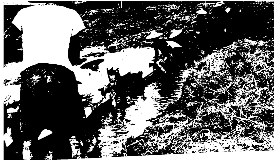
Men cut the heavy clay, women slide it up the ramp to make embankments and causeways. The place is Hong Kong ; the purpose, to build ponds for the cultivation of fish, a rich source of food
