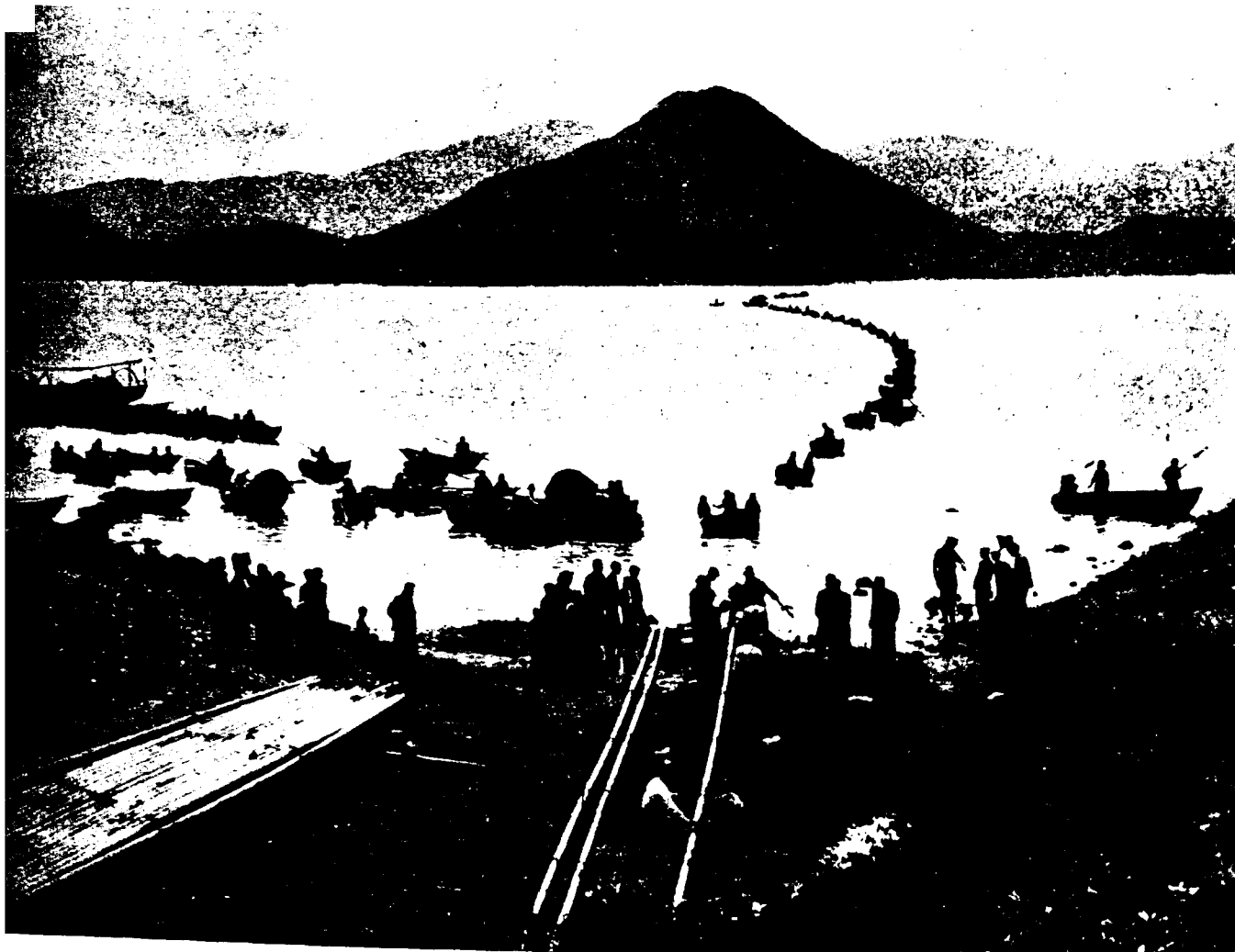
Fishermen on the island of Kat O, off the north-east coast of Hong Kong, help to lay a 22,000-foot-long pipeline to bring fresh water from the mainland. Organised by British Army engineers, 130 sampans carried the three-inch diameter pipes beneath their hulls. The 120-foot lengths were joined at sea and then, at a prearranged signal, the fishermen pulled slip knots and the pipeline fell to the seabed
