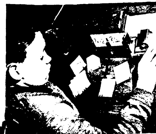
COMPARATOR MACHINE. The boy is pressing a lever after inserting a card with his answer to the problem. A correct answer causes a light to flash. No light flashes for an error, which is recorded.
