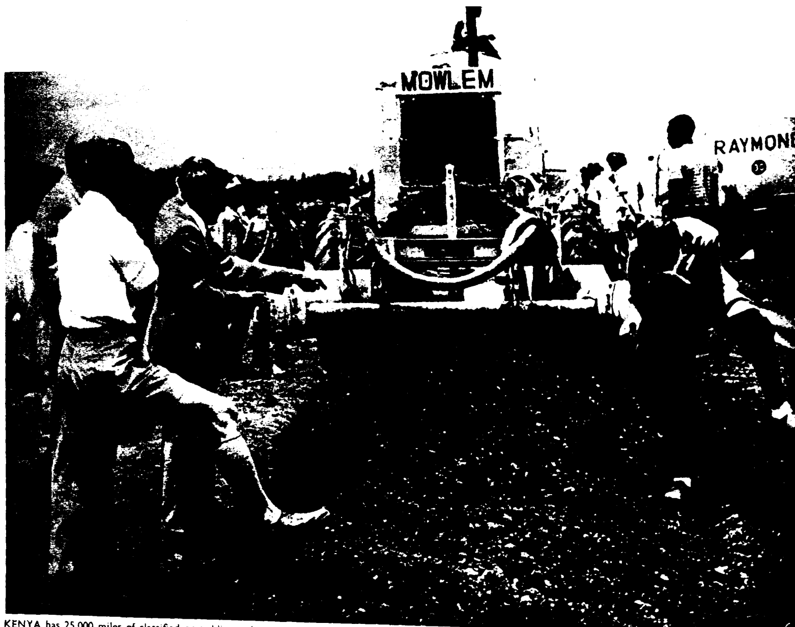
KENYA has 25,000 miles of classified or public roads, not all well surfaced. Great progress is being made providing old roads with better surfaces and building new roads. Above: This machine at work on the road from Nairobi to Nyeri mixes cement with soil to produce stabilised soil on which a bitumen surface can be put down. Below: A study in concentration as Kenyans who met to discuss the problems of soil stabilisation, in Nairobi in 1960, inspect a newly made hard surface on the same Nairobi to Nyeri road. This road is now well surfaced over its entire 96-mile length.
