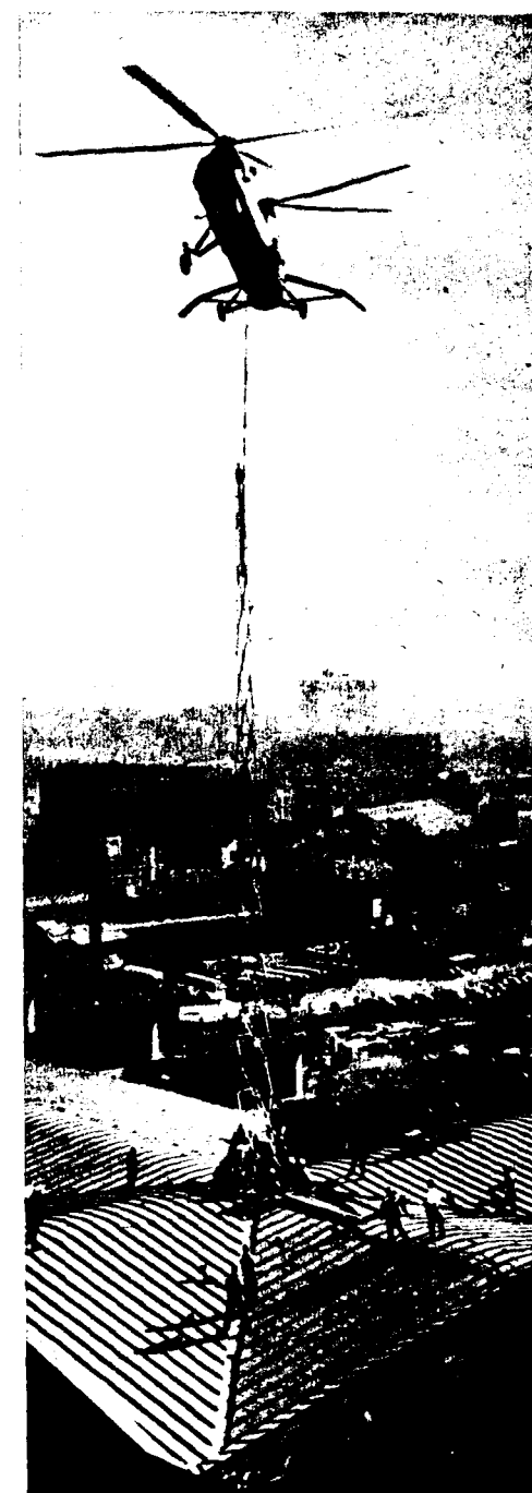
THE finishing touch (above). A twin-rotor "Belvedere" helicopter of the R.A.F. gently lowers a 78-foot metal lattice spire on to a base plate one yard square, on the roof of the cathedral.
