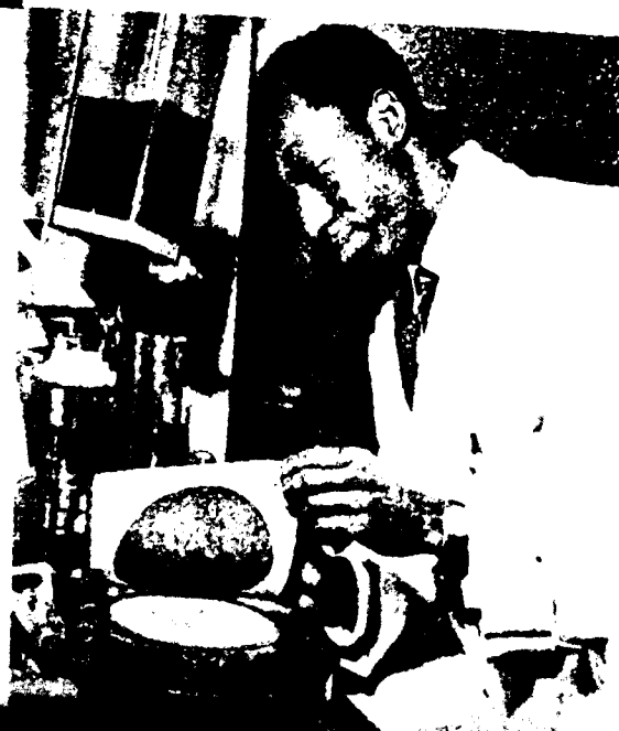
MR. J. O. RITIBI, from Ekiti in Western Nigeria, removes a sample of standard sheet from the grid of a paper-making machine. Nigeria is producing paper of her own for the first time.
