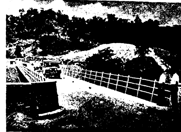
OPENING a road bridge. Road development in Tanganyika includes the building of a grid of four trunk roads from north to south and three from the coast westwards.
