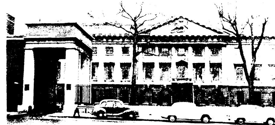
THIS is the Mint, an imposing building facing the Tower of London. In addition to its normal commitments it is now producing 1,000 million coins for the Federation of Nigeria.
