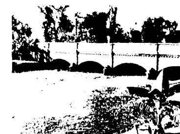
A CANAL and bridge in Pakistan. New canals will stretch 400 miles.
