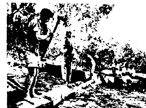
THIS kereti log is being squared, ready to be sawn into planks. They were for nine homes, built for a Housing Society.
