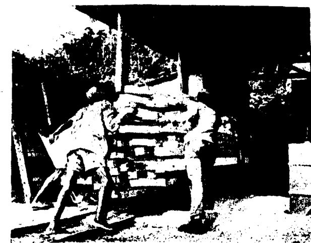
TIMBER is put into a special plant near the sawmill (left), which makes it both insect-proof and rot-proof. Pine, which is now being planted at Shume, can be impregnated more easily than other softwoods—Cypress and Cedar—which grow in the region.
