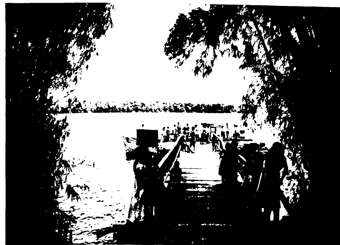
A substantial wharf, or stelling, the completion of which was largely due to the inspiration and drive of young Colin Henfrey. It was opened by the Governor of British Guiana, Sir Ralph Grey.
