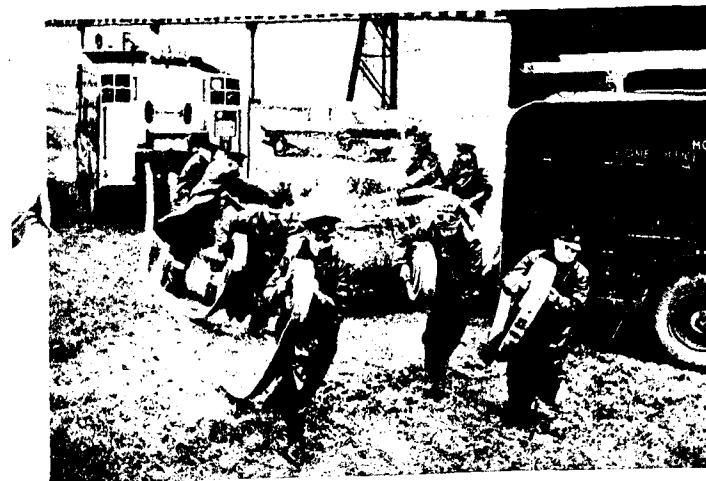
NEW USES FOR MODERN FABRICS. One hundred and twenty 2,500-gallon Neoprene-coated water tanks have been ordered by the United Kingdom Home Office for emergency use by Britain's Fire Services. This one is being demonstrated at a training centre in Gloucestershire. The tanks are light, cheap, easy to put up, and rot-proof, enabling them to be stored without damage.
