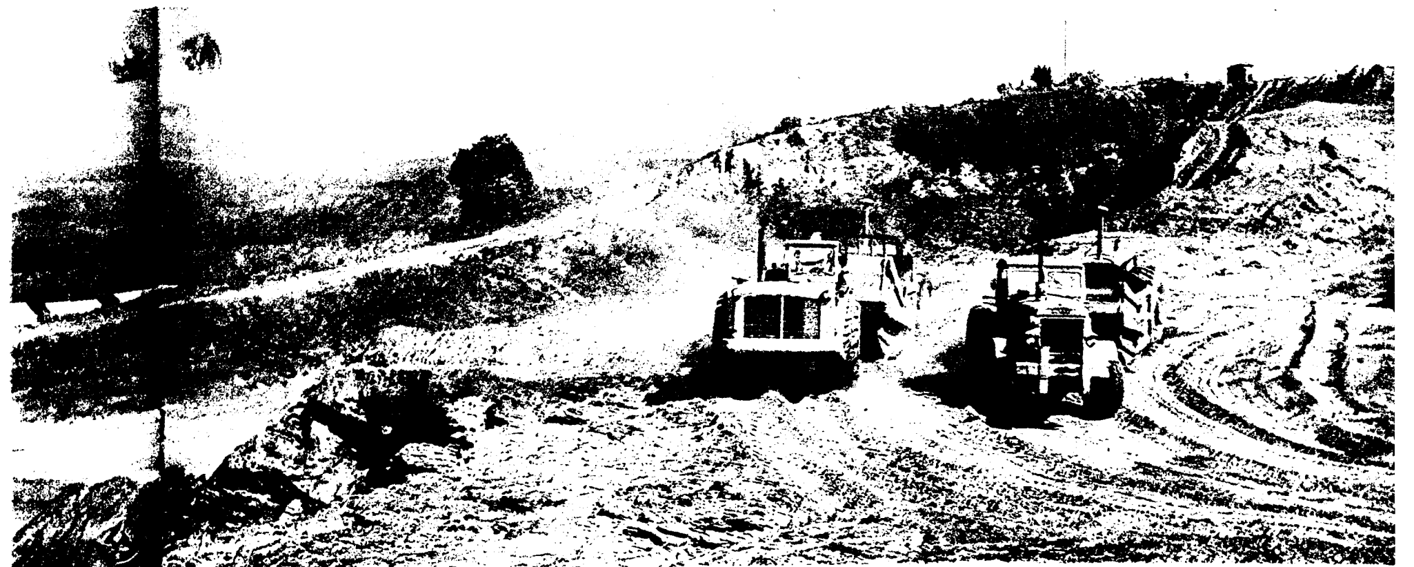
TWIN power scrapers, like busy insects, gather iron ore from the Masaboin iron mine at Marampa. In 1958 Sierra Leone exported nearly 1½ million tons of crude iron ore worth £4,490,460.
