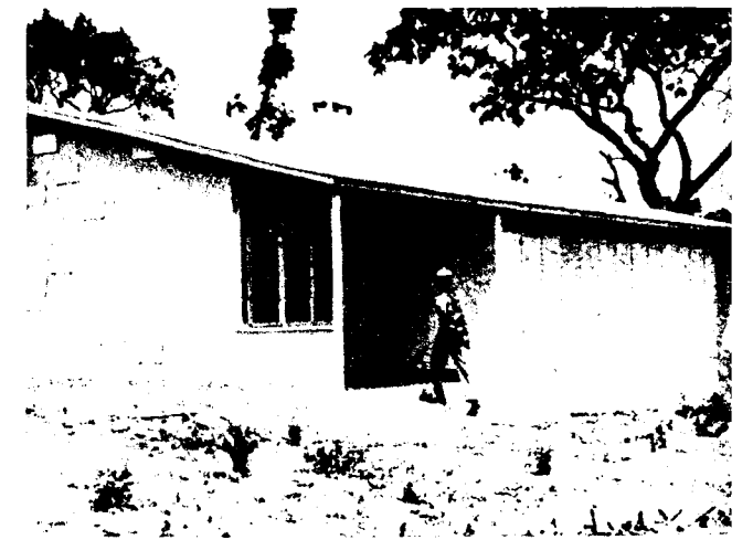
THE SMALLEST type of house on the estate—700 sq. ft., for £1,000. This includes the cost of the plot, sewerage, water and road development.
