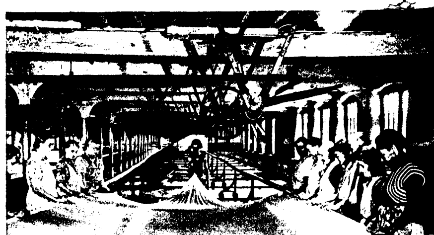
WORKERS in a dressing and dyeing works stretch a length of lace across a flat frame in order to set the lace to its correct width and length. Nottingham has made a tablecloth 35 ft. long.
