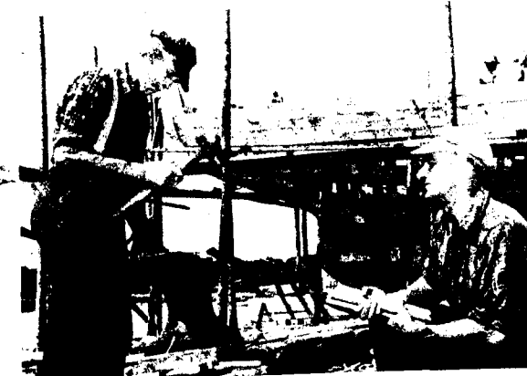
SHIPWRIGHT Alton L. McKay (above) marks out the forward end of the pilot house for a wooden ship being built at Shelburne, Nova Scotia. Below: Another Nova Scotian, George Acker, cuts bolts for use as fastenings.
