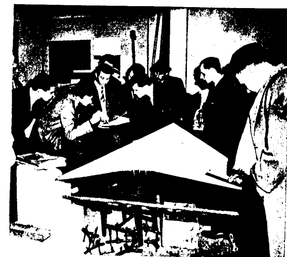
A NEW SYSTEM of concrete stressing was explained to the visiting Canadians at the Cement and Concrete Association's structures laboratory at Fulmer, Buckinghamshire. The Association provides a free technical advisory service.
