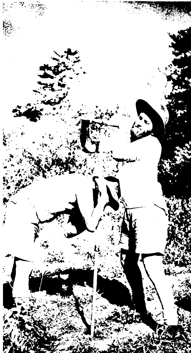
PROBING (above) to measure the depth and nature of deposits near the main excavations. The instrument in use—called an earth auger—can reach a depth of 25 feet. Right : Members of a working party use a surveyor's level to locate the position of an excavation.
