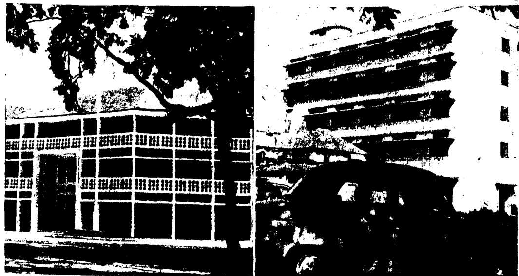
NEW PUBLIC BUILDINGS. The facade of new Government offices in Dar es Salaam, the capital of Tanganyika, contrasts with the simplicity (right) of the first complex section of the new Post Office at Suva, Fiji. From F. D. de Souza, P.O. Box 2828, Dar es Salaam, Tanganyika. And: M. Lal, c/o G.P.O., Suva, Fiji.
