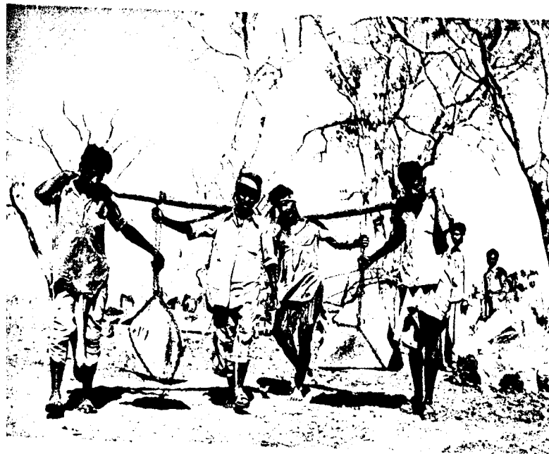
WOMEN , as well as men, carry stone to the construction site. Much time and expense were saved by working without special equipment and machinery.
