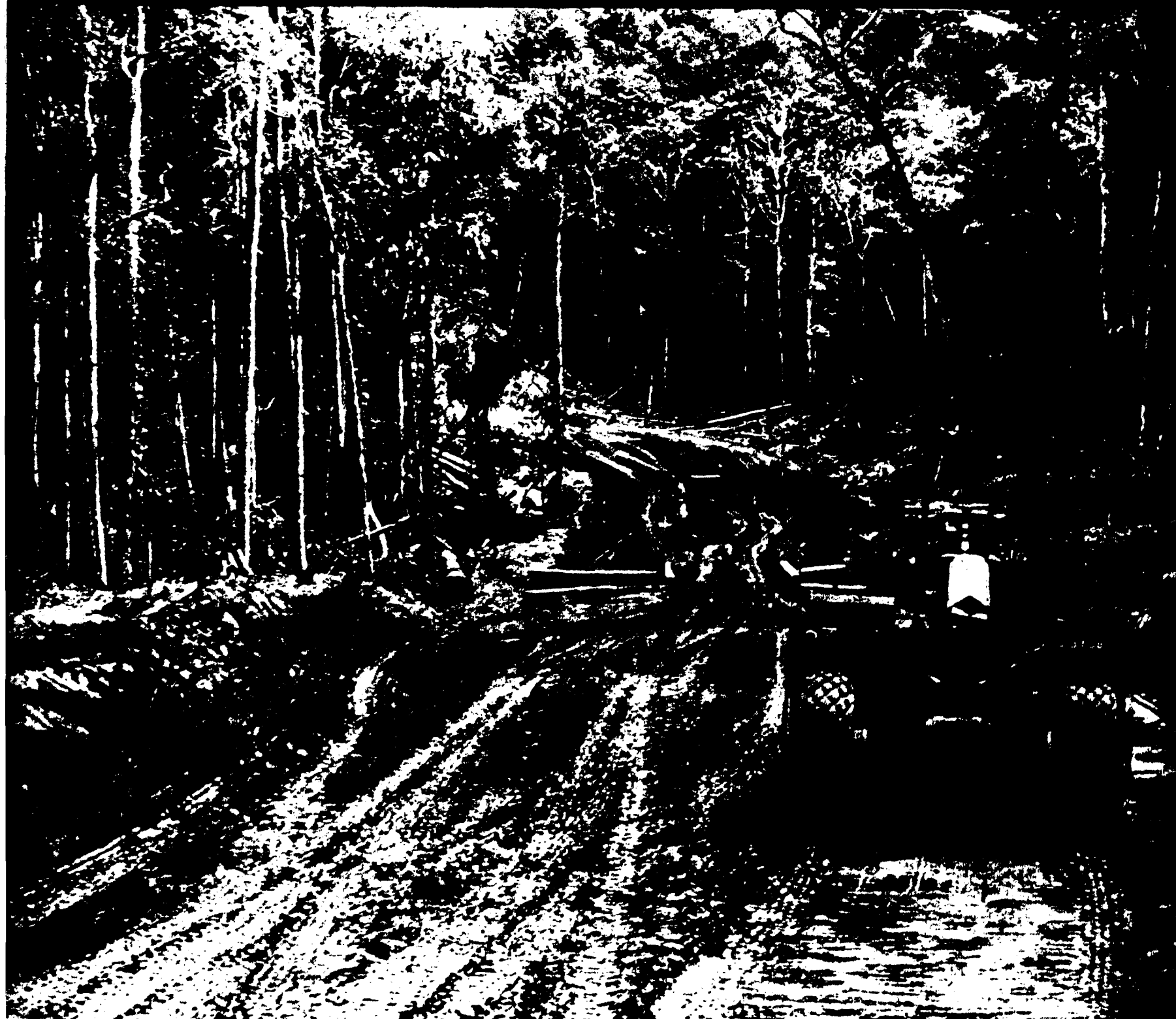
MALAYANS and troops from the United Kingdom, Australia and India, worked together to build this road through thick jungle in the State of Kedah.
