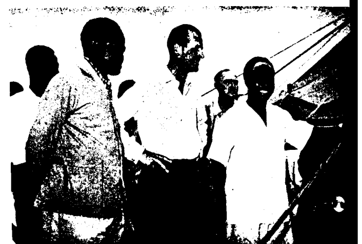
AT SHAI HILLS quarry, which provides rock for the Tema Harbour breakwaters. Besides the deep-water harbour, costing about £18 million, Tema will have a new township and an industrial area.
