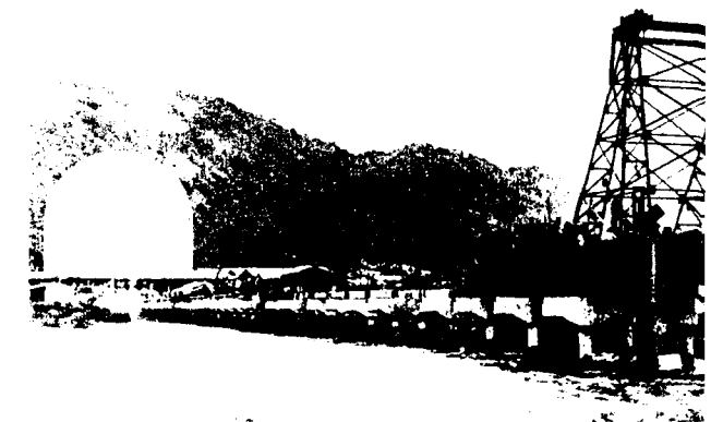
WORK goes ahead on the 3,280-foot-long jetty at Trombay, built by Cementation Co. Ltd. in association with the Patel Engineering Company of Bombay. It cost $624,000. Both companies, as a joint venture, built the reinforced pump house. Constructed in a dry dock in Bombay Harbour, it was towed into position at the head of the jetty—a distance of 12 miles. Value of the contract, £180,000.
