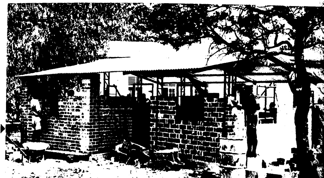
A TEAM of four unskilled labourers put up the frame and roof of one of these houses in three hours. Individual components are extremely light in weight.
