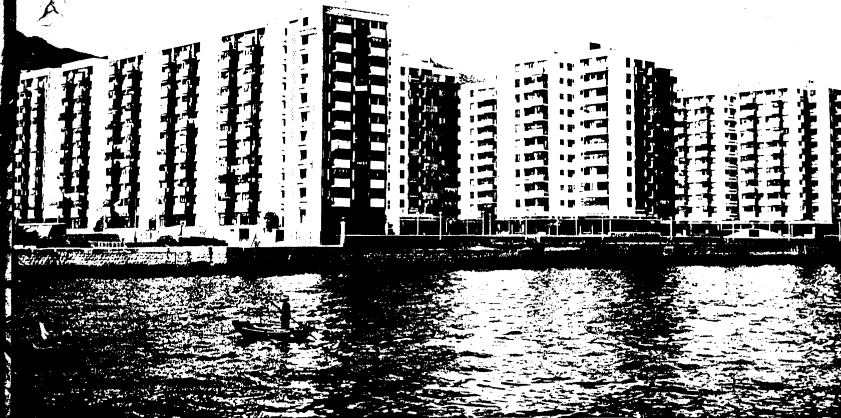
THESE FLATS, completed in 1958, house several thousand people; they pay a rent ranging from $4 14s. to $10 12s. a month, which is inclusive of rates.
